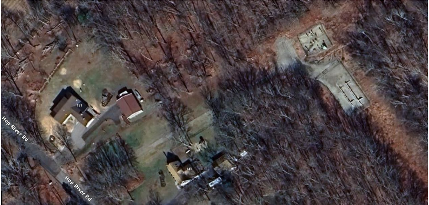
Existing Tap Site on E-1 pipeline system
