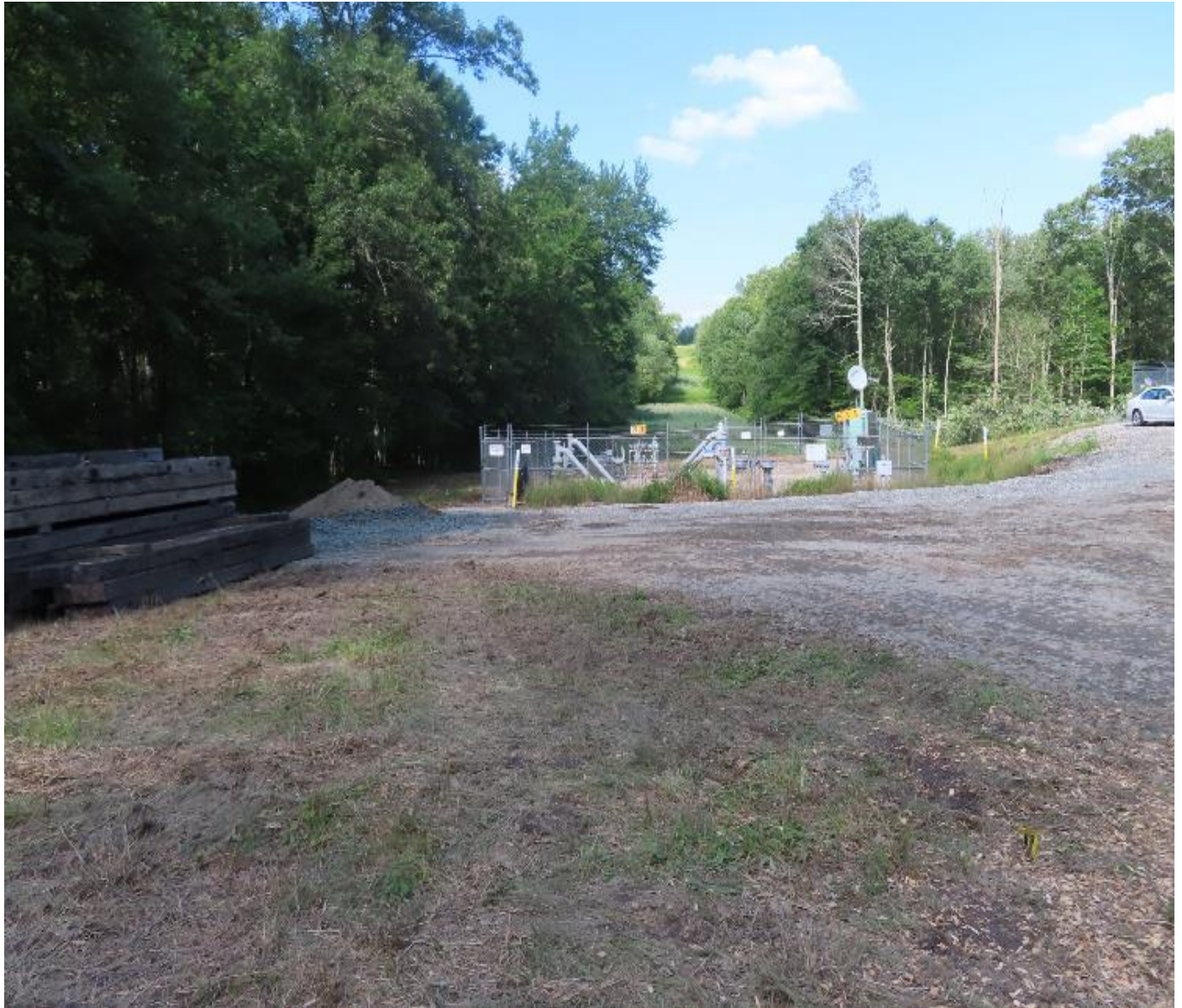
Photo 4. View (looking northeast) of fence valve station where 30-inch valve will be replaced.
