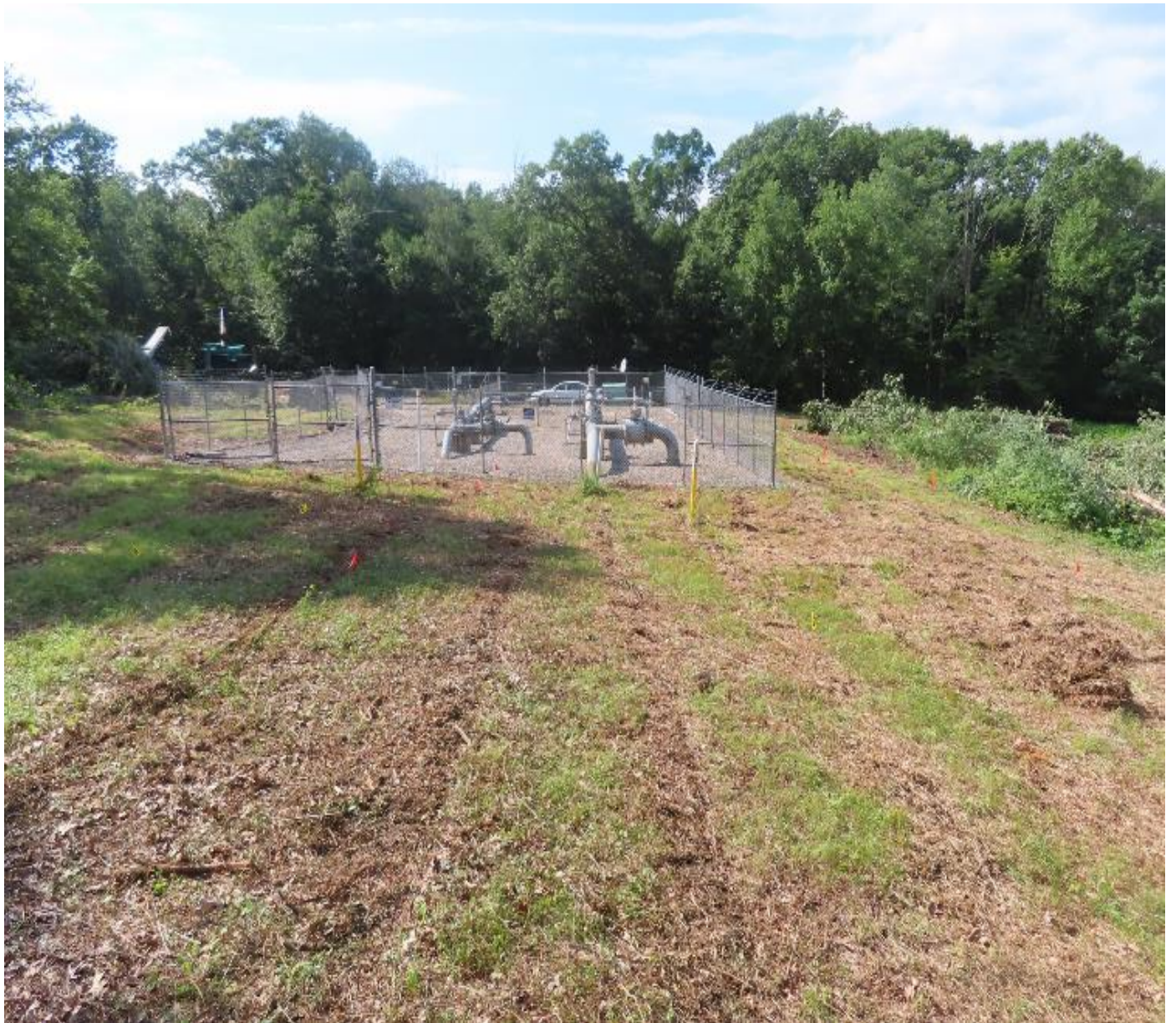
Photo 8. View (looking northwest) of E-System easement after mowing.
