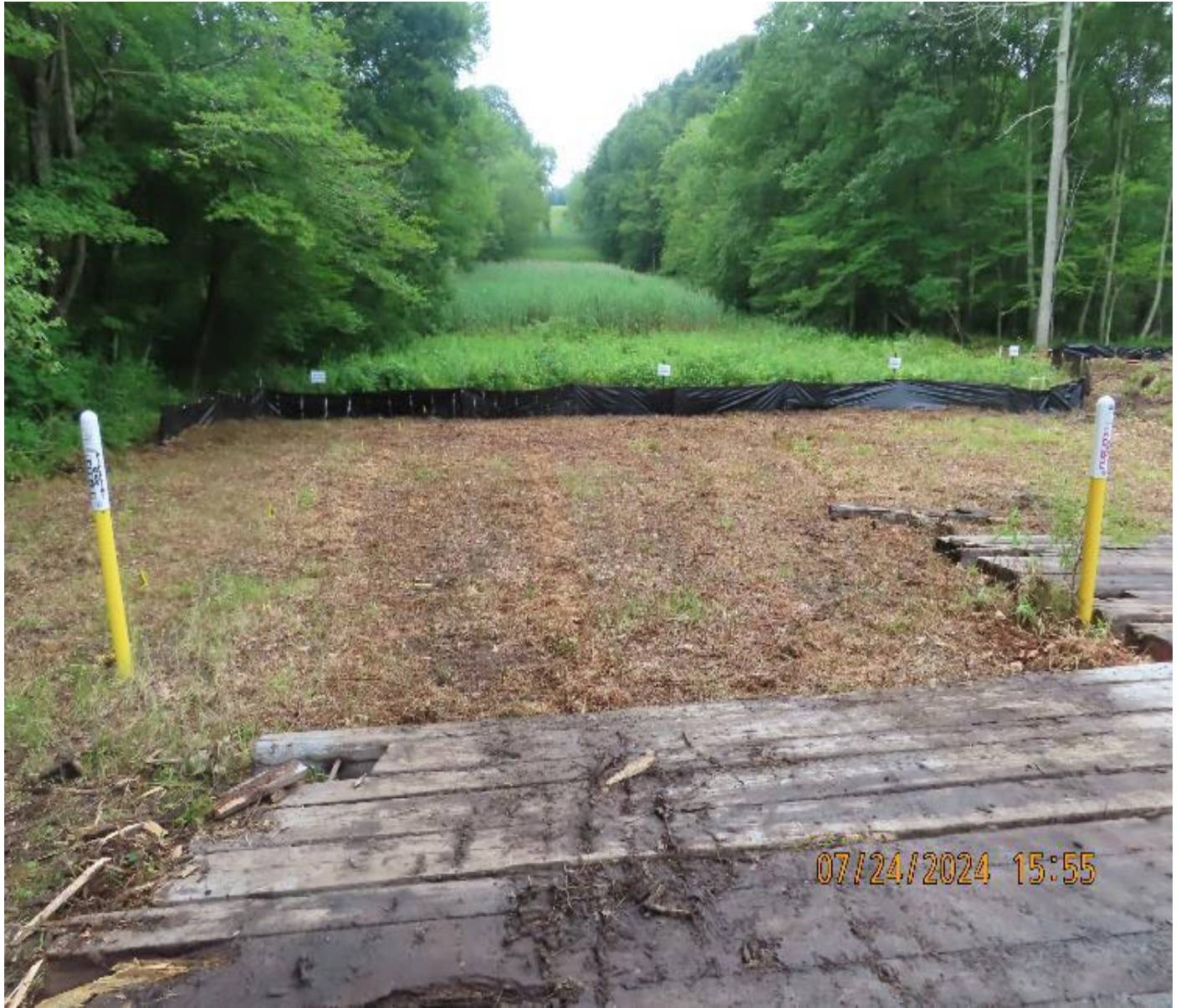
Photo 6. View (looking northeast) of silt fence, wetland signage, and vegetative buffer along northeast site boundary. Mowing has occurred in this area but no ground disturbance.
