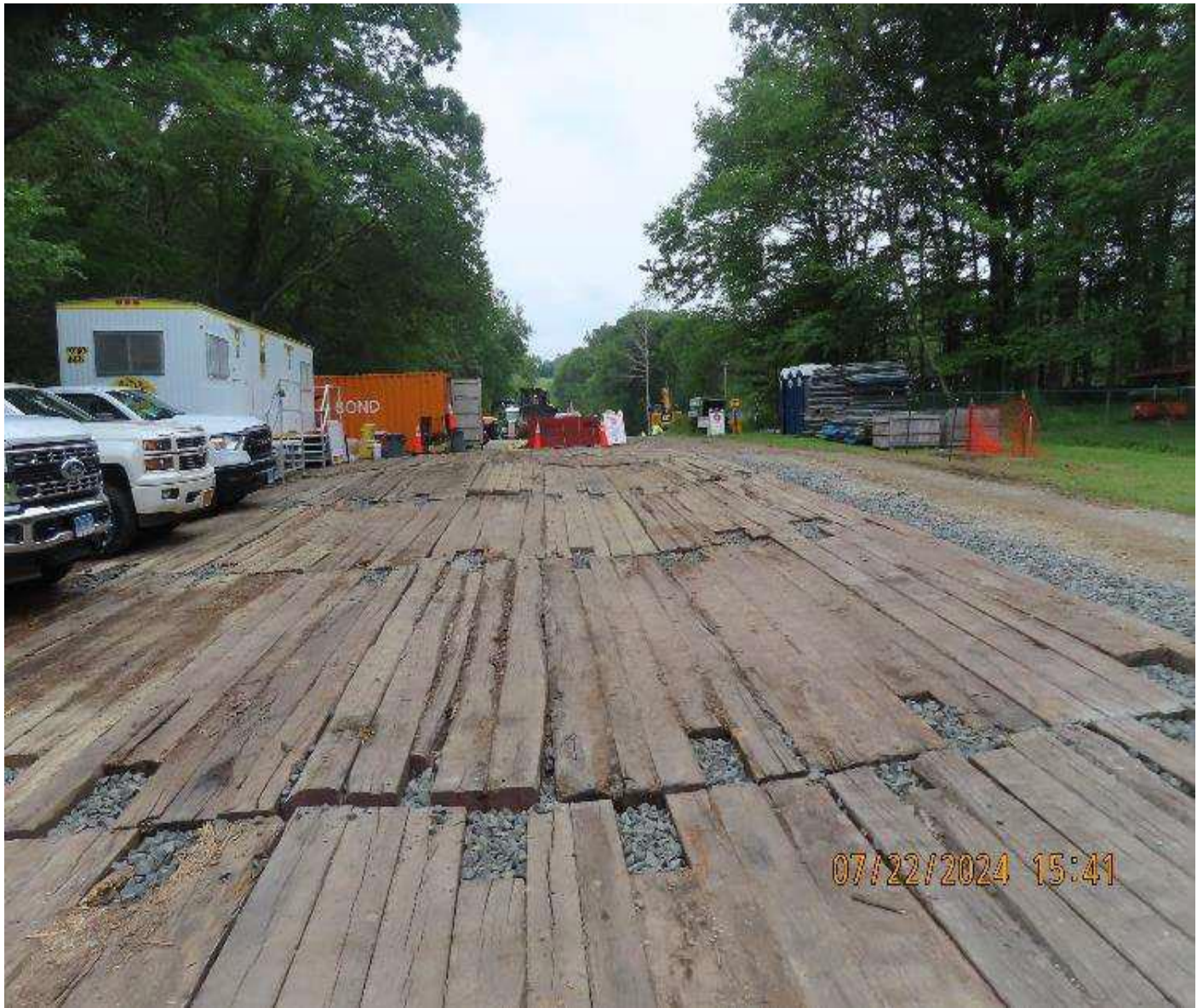
Photo 1. View (looking northeast) of matted staging area for job trailers and vehicle parking.
