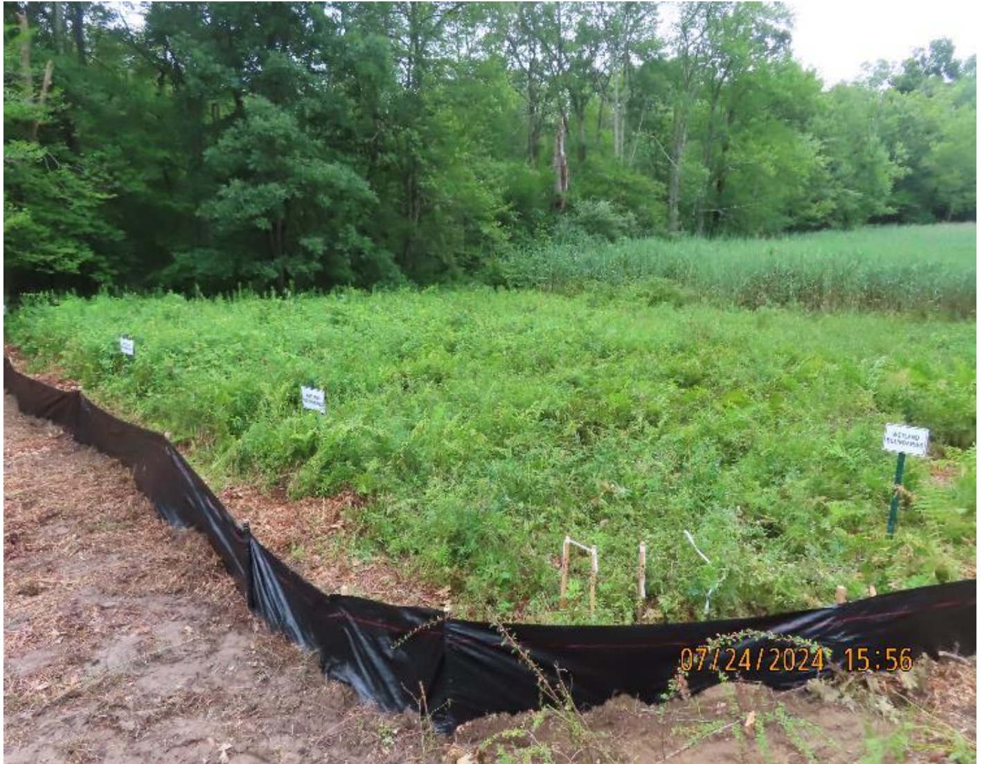
Photo 5. View (looking north) at silt fence, wetland protection signage, and vegetative buffer for wetland W-CZ-01.
