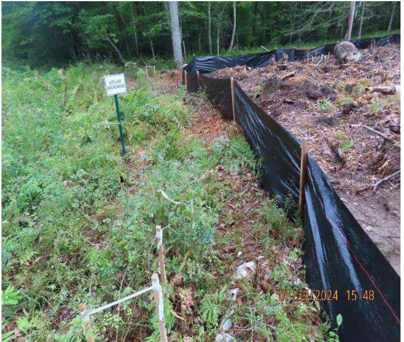
Photo 7. View (looking northeast) of silt fence perimeter near wetland W-CZ-01.
