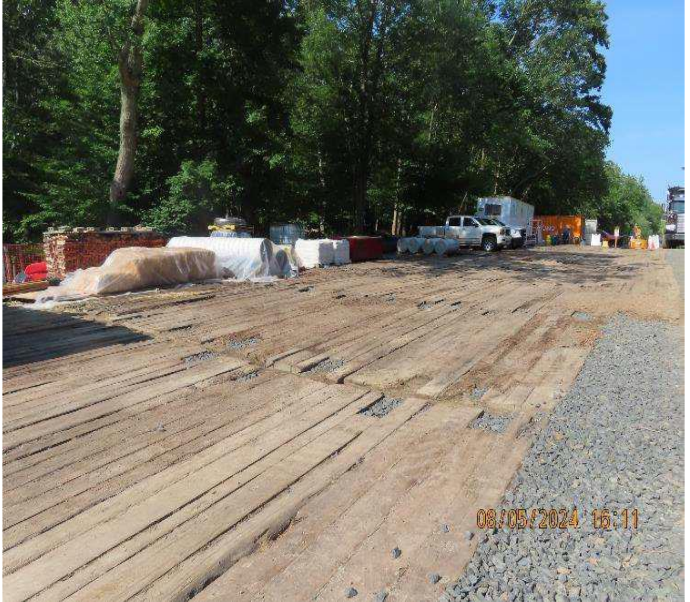
Photo 2: View (looking northeast) of staging area.
