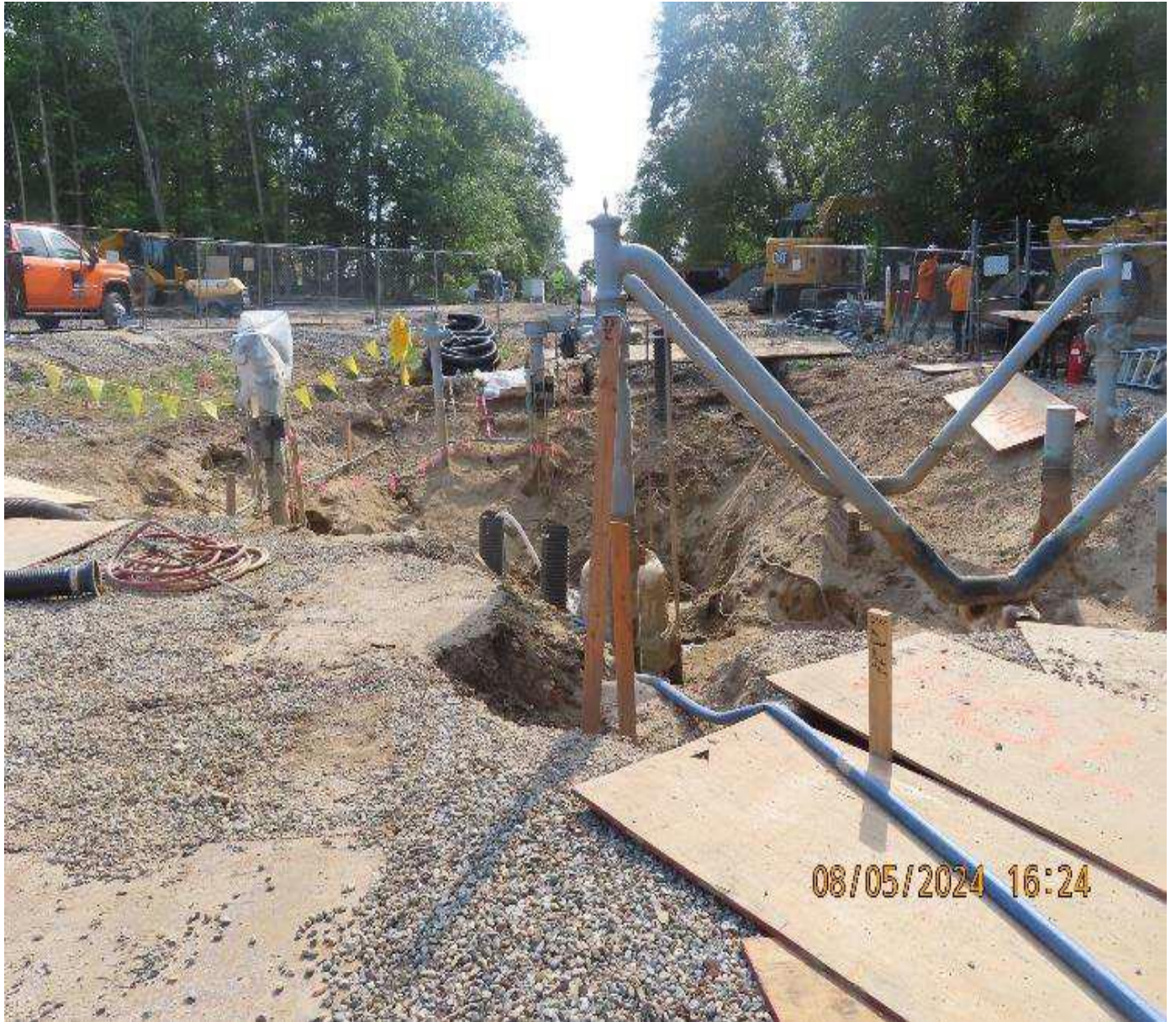
Photo 5: View (looking southwest) of excavation work in valve yard.
