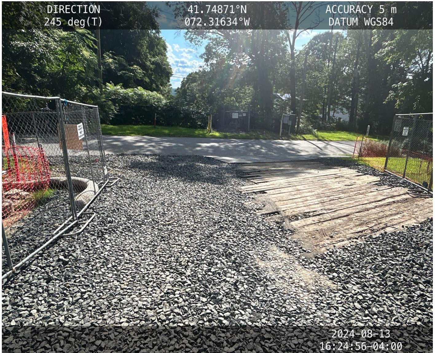
Photo 2: View (looking southwest) of entrance from Hop River Road.
