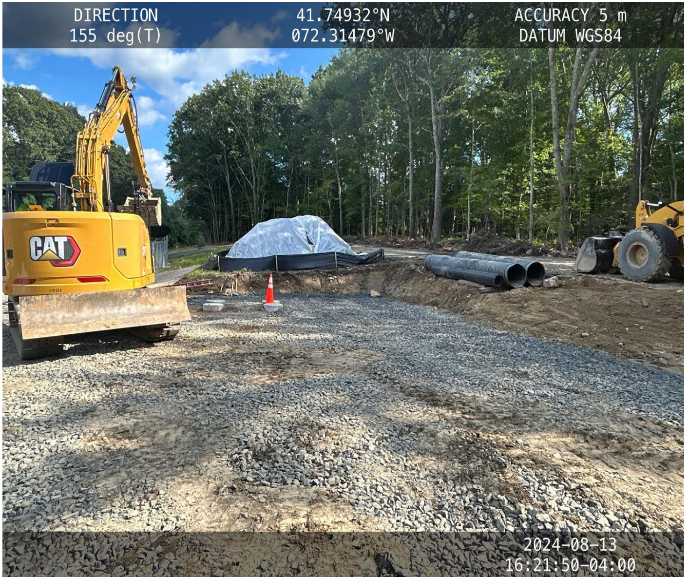
Photo 6: View (looking southeast) of soil stockpile covered and surrounded by perimeter ECDs.
