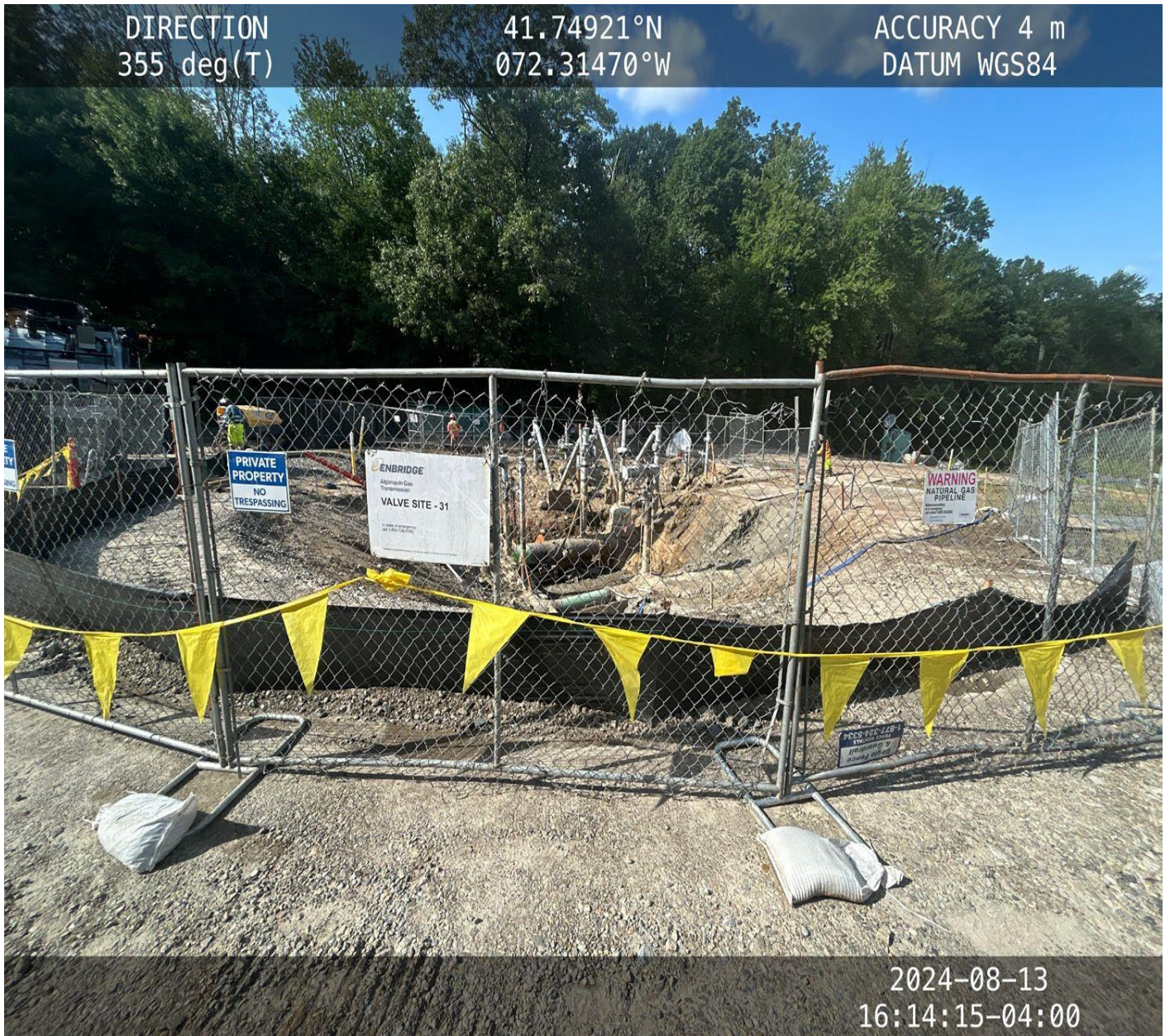
Photo 4: View (looking north) of excavation progress in valve yard.
