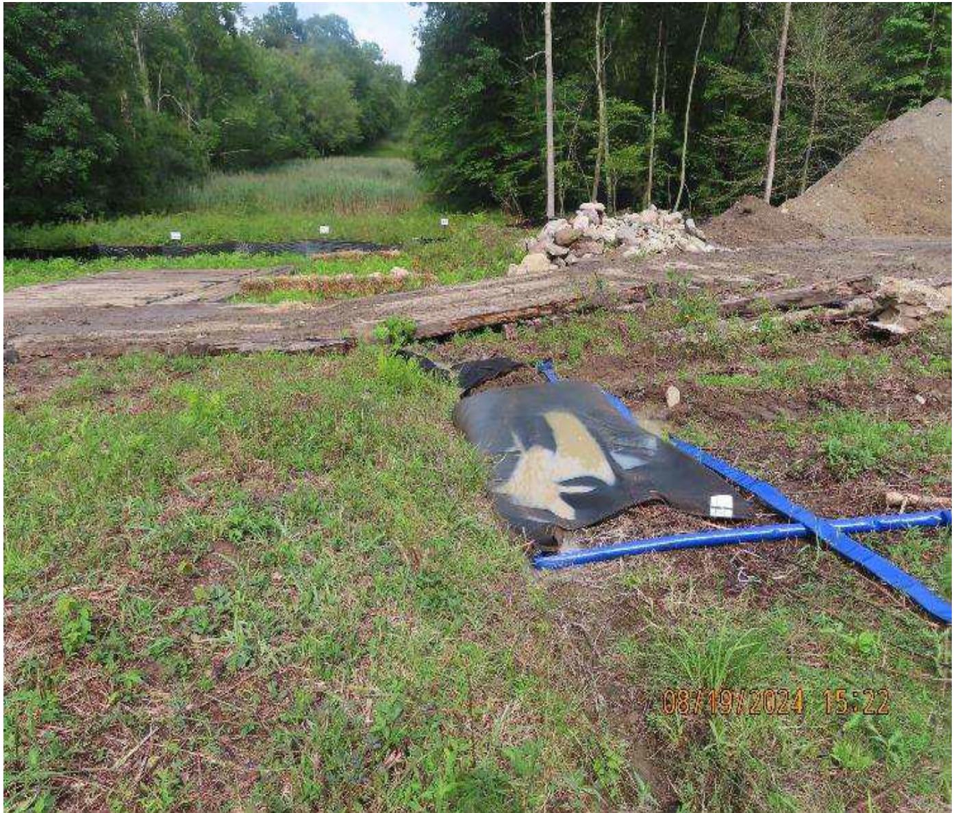
Photo 4: View (looking northeast) of excavation dewatering through filter bag.
