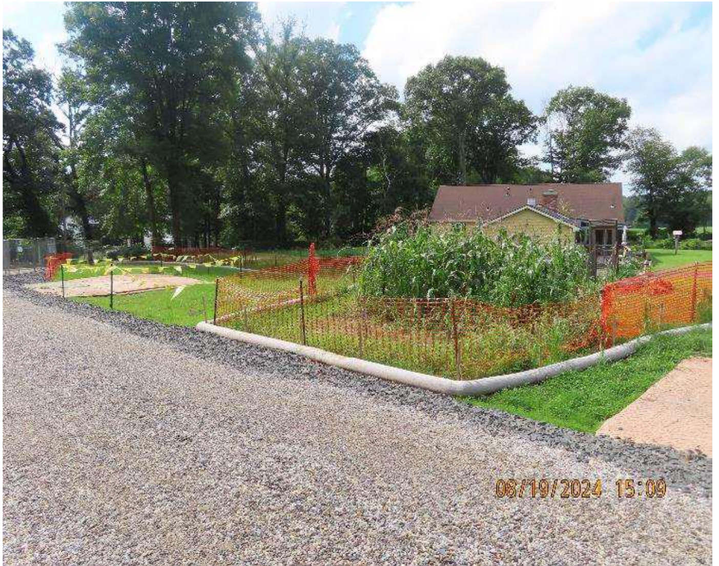
Photo 1: View (looking west) of perimeter controls protecting nearby residences.
