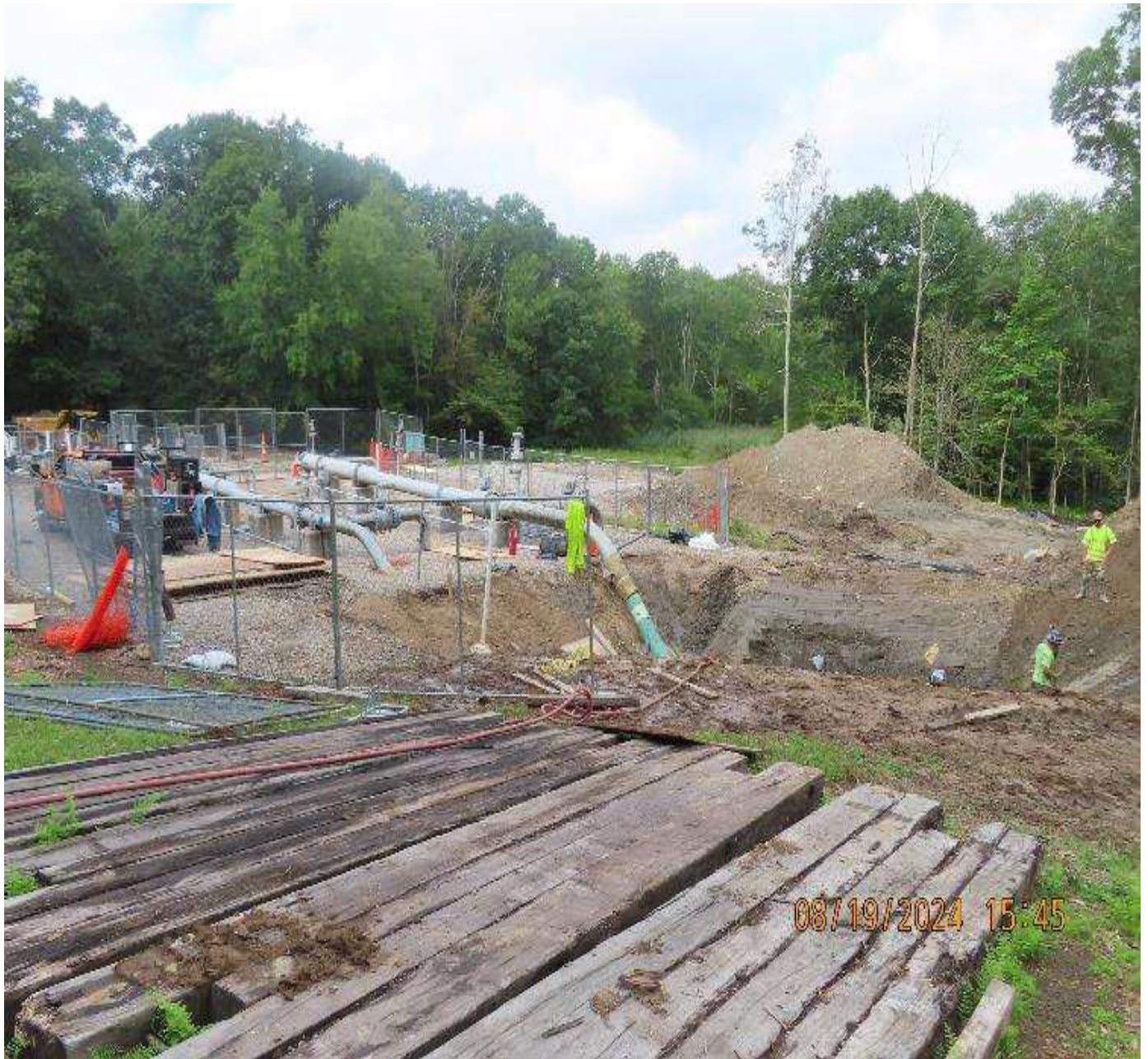
Photo 6: View (looking north) of tie-in excavations for E-1 and E-1L.
