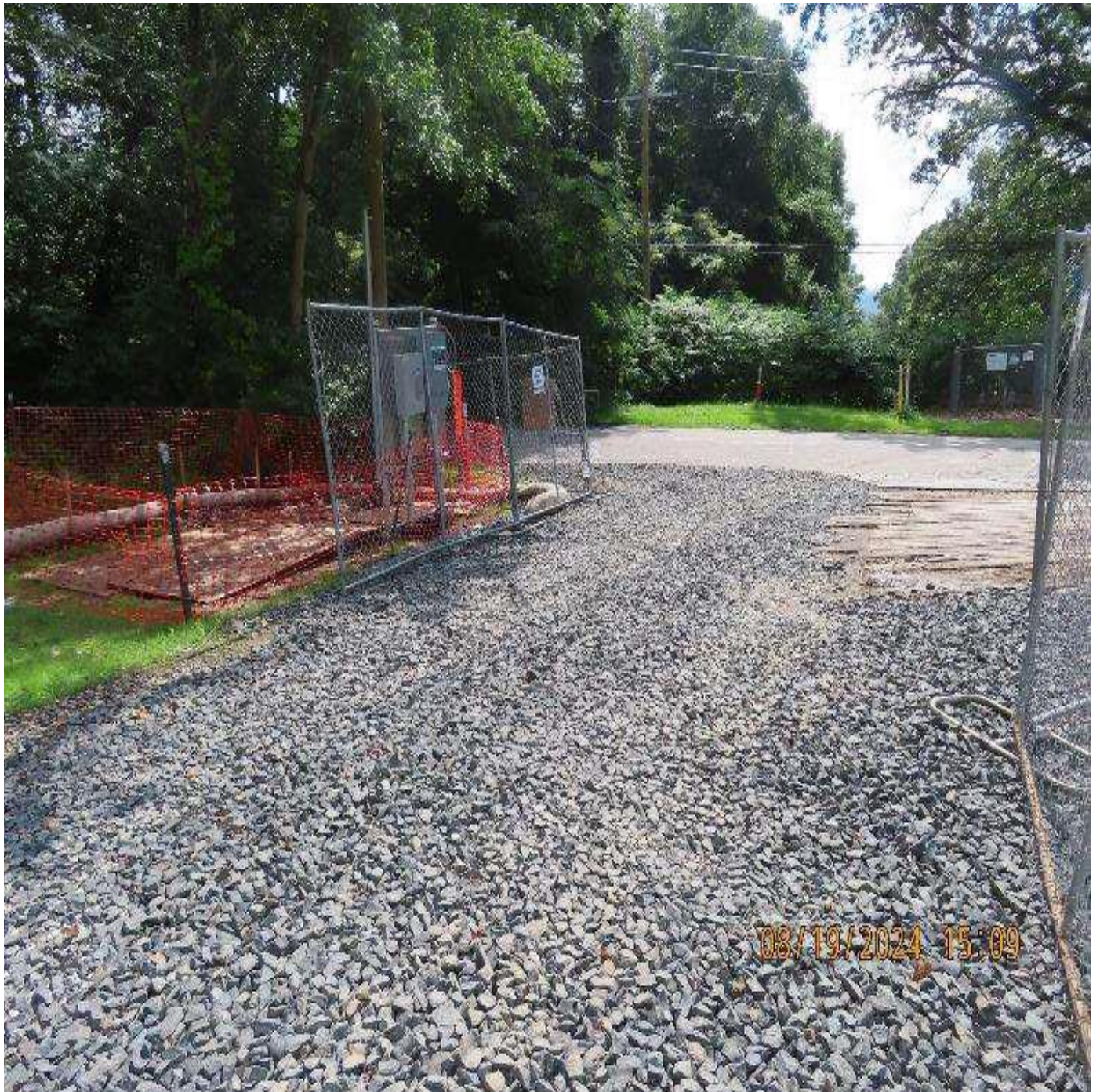
Photo 2: View (looking southwest) of construction entrance from Hop River Road.
