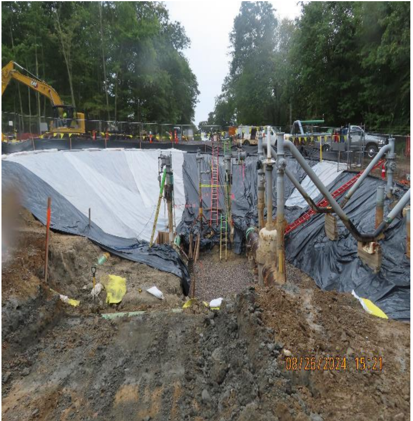
Photo 2: View (looking southwest) at excavated areas in the valve yard.
