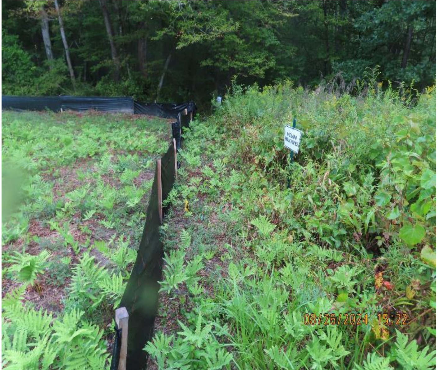
Photo 3: View (looking northwest) of perimeter SESCOs, vegetative buffer, and signage protecting wetland area.
