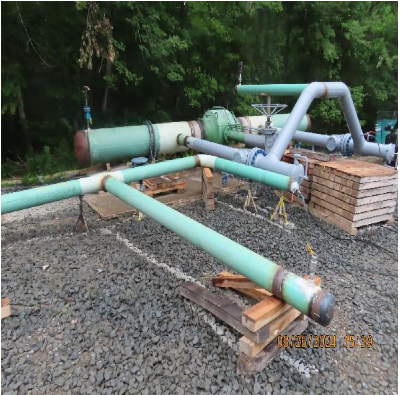
Photo 7: View (looking west) of new piping infrastructure ready for hydrostatic testing.
