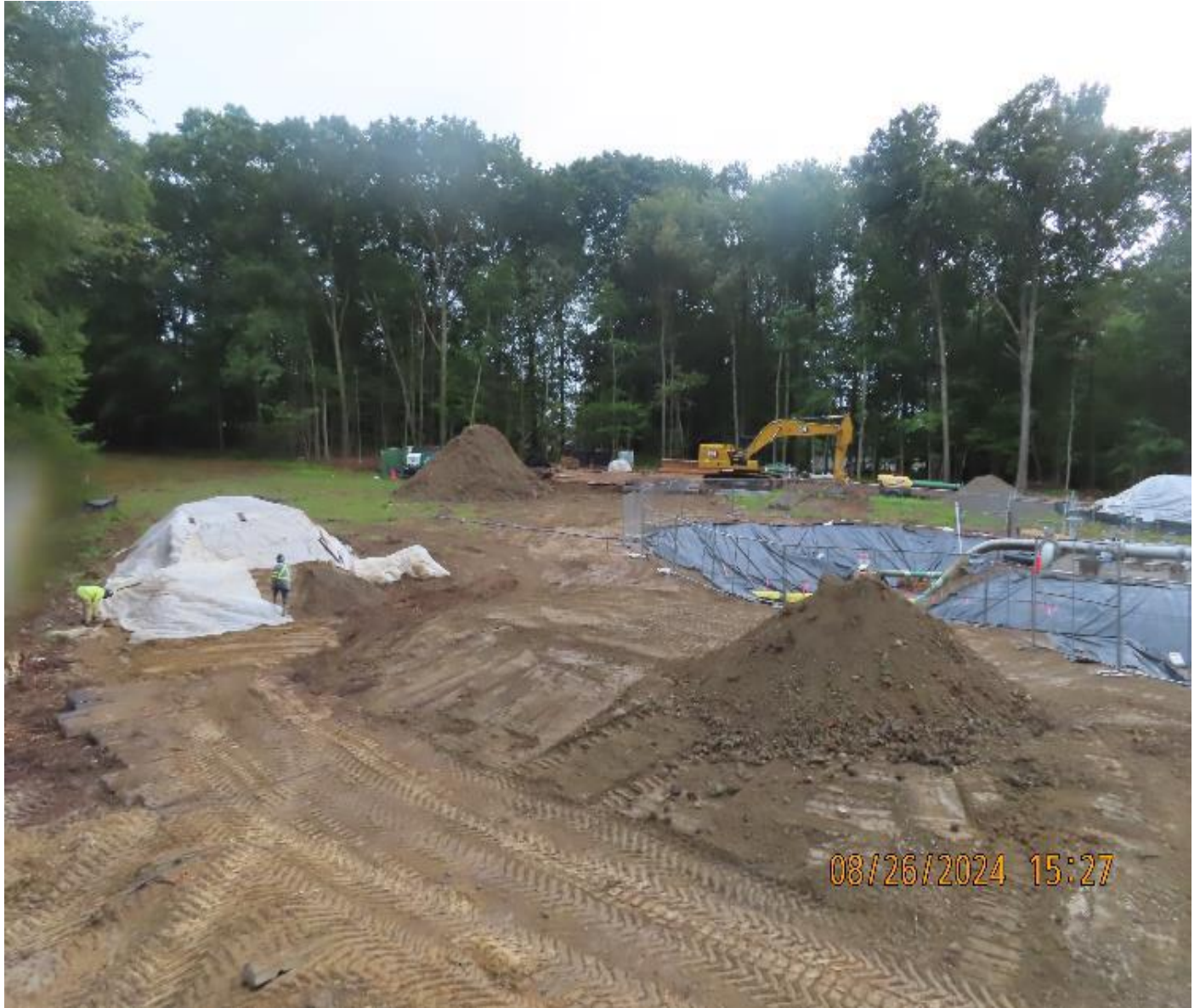
Photo 4: View (looking south) of southeastern portion of site showing stockpiles being covered at the end of the workday.
