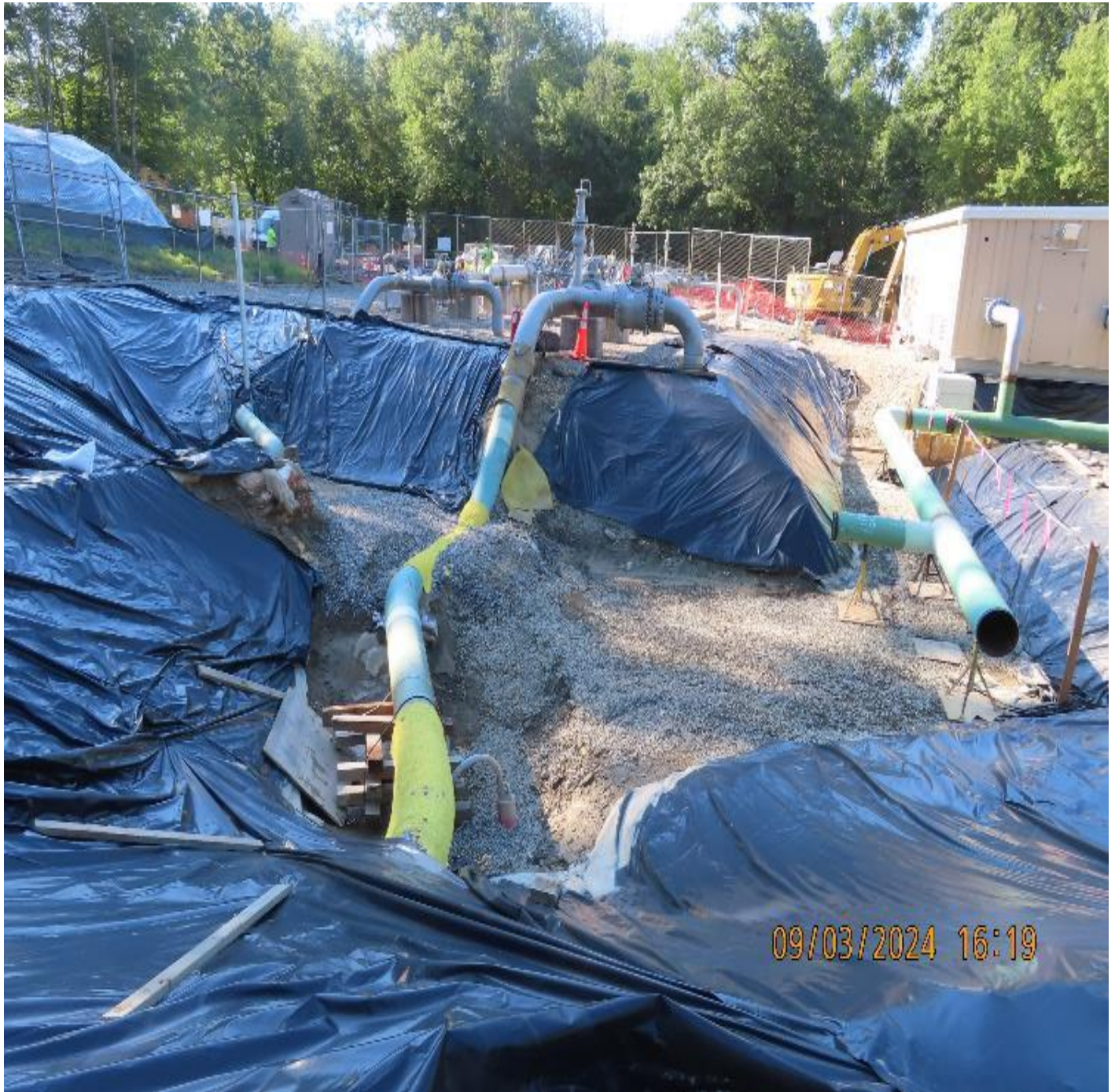
Photo 3: View (looking northwest) of excavation for E-System piping tie-ins.
