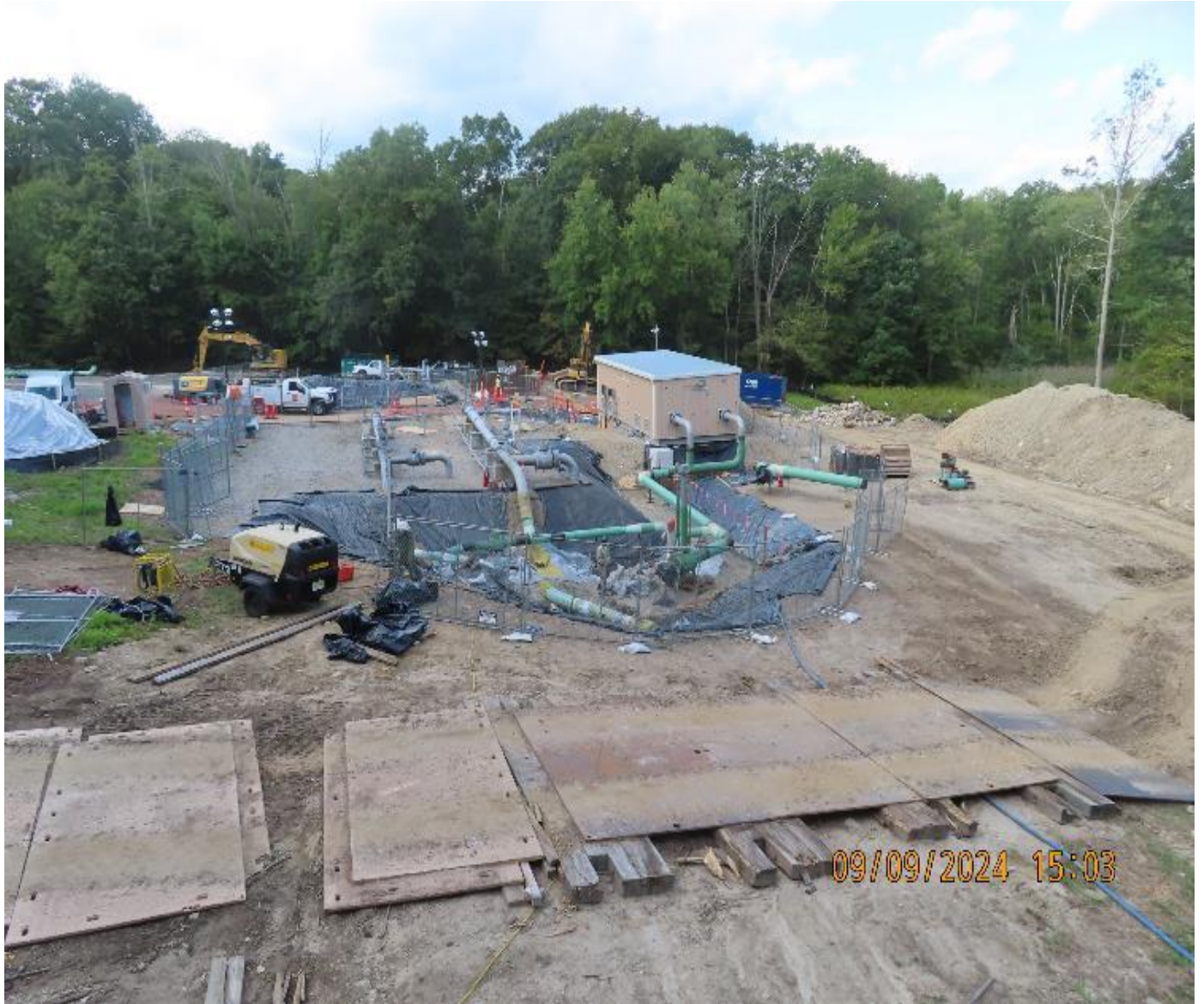
Photo 7: View (looking northwest) of construction work in valve yard.
