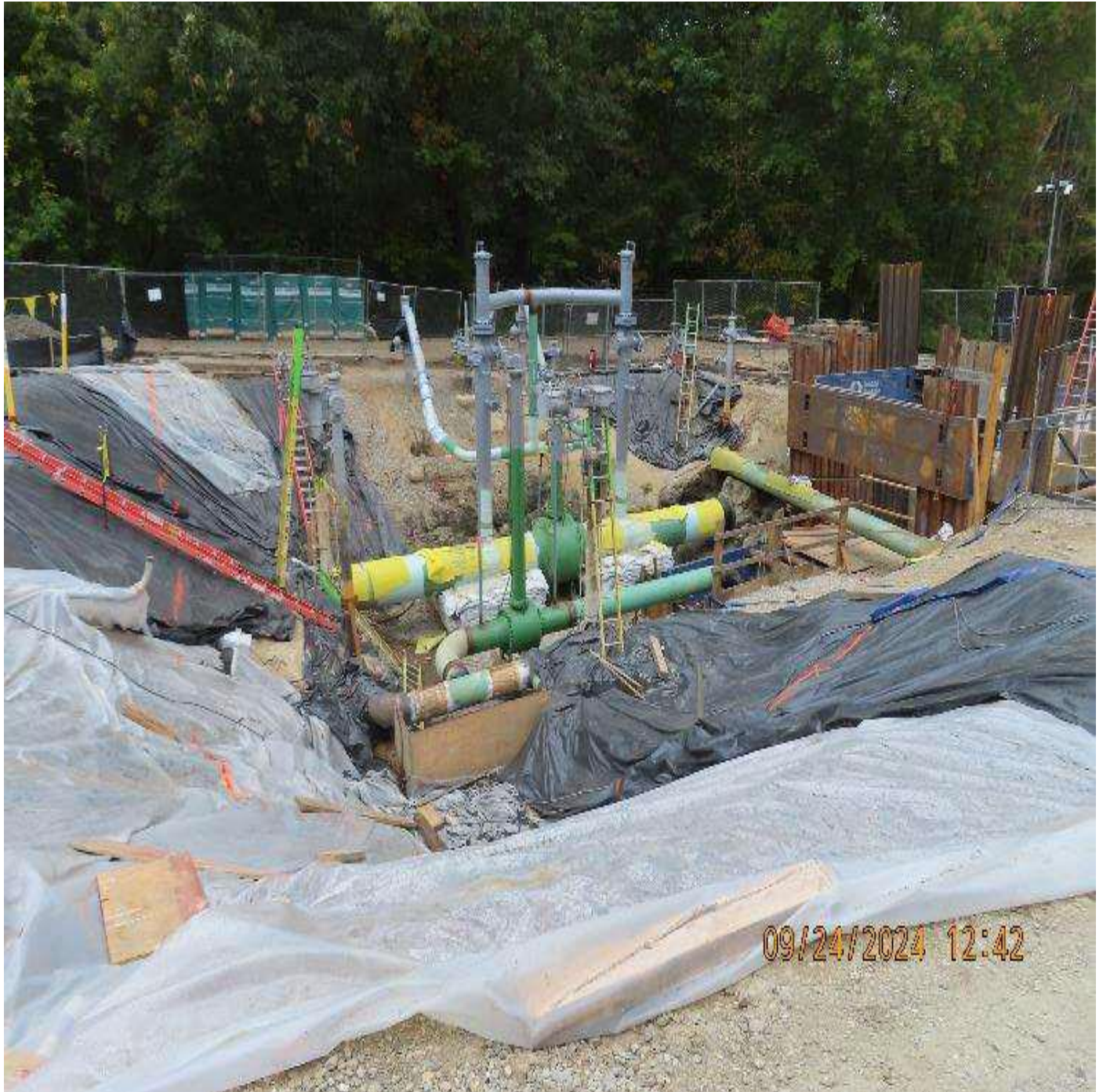
Photo 6: View (looking northwest) of mechanical work in the valve yard.
