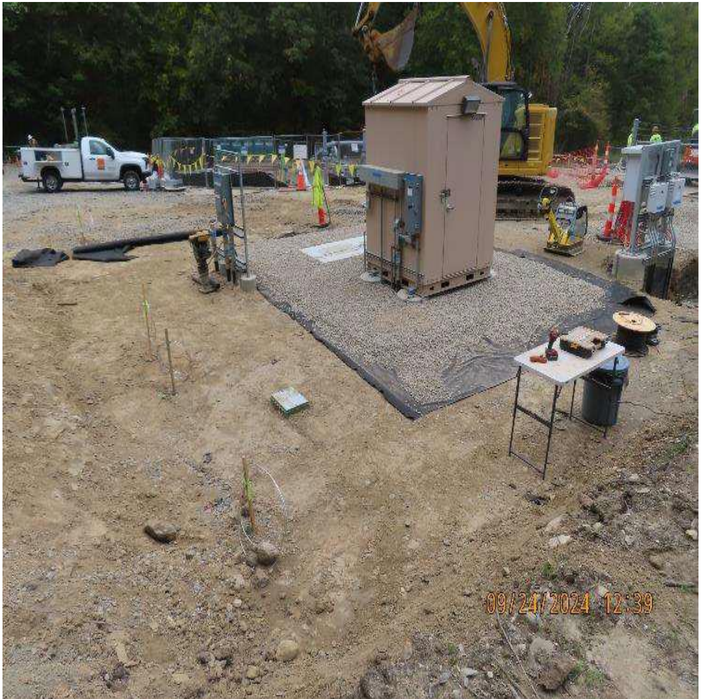
Photo 7: View (looking northwest) of stone surfacing around new RTU building.
