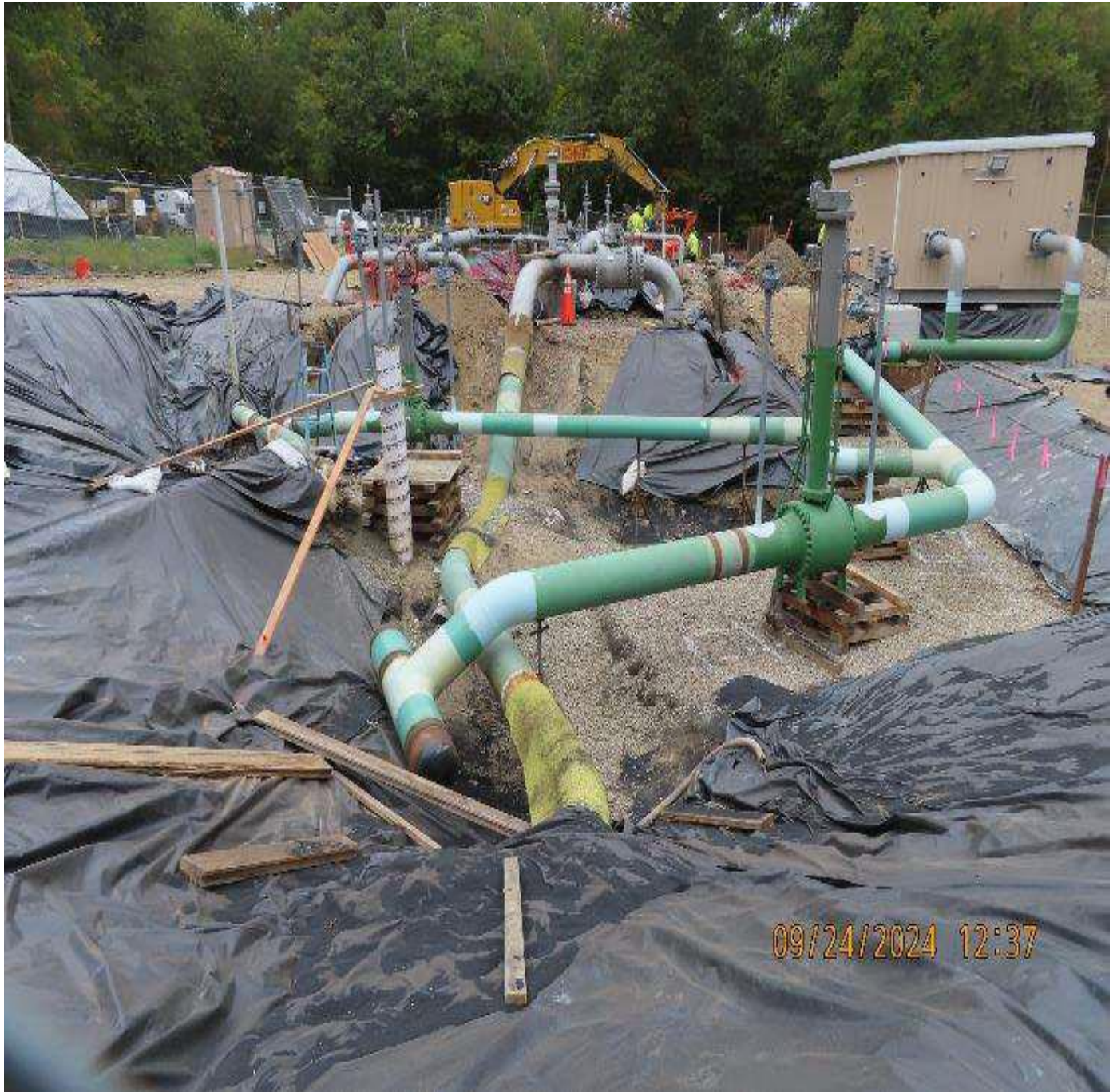
Photo 5: View (looking northwest) of mechanical work in the valve yard.
