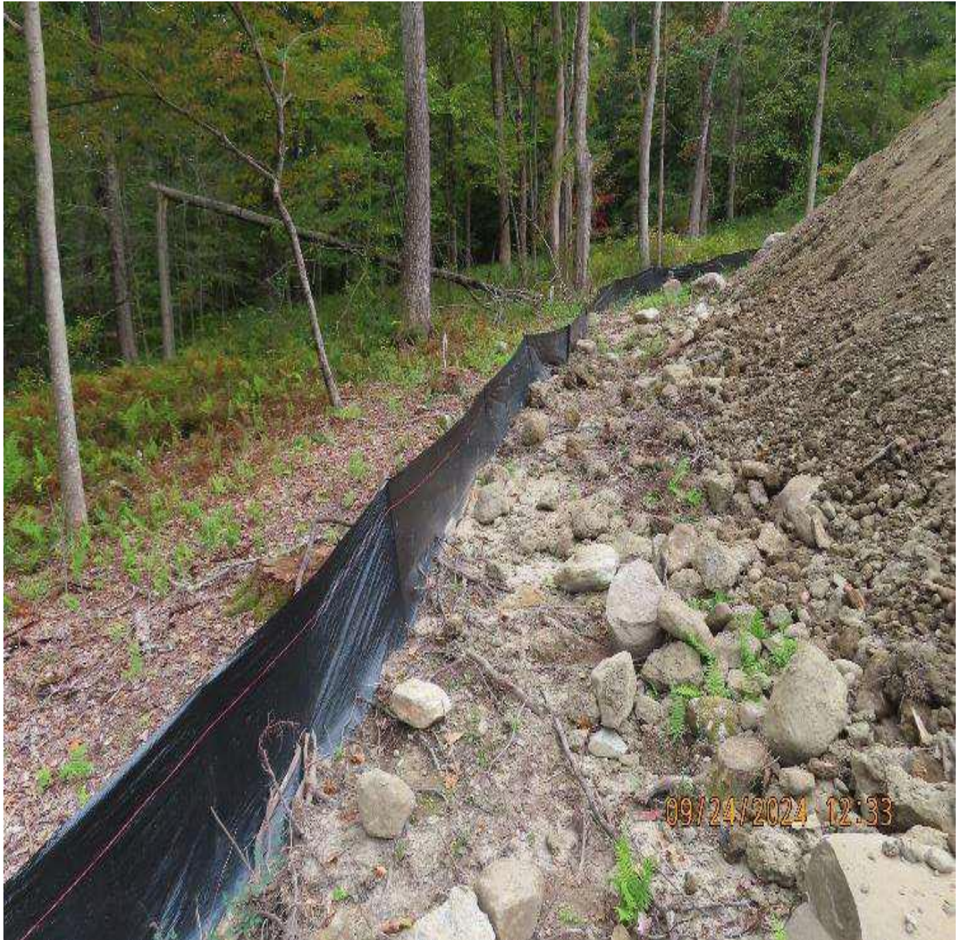
Photo 4: View (looking southeast) of ECDs along backside of excavated soil stockpile.
