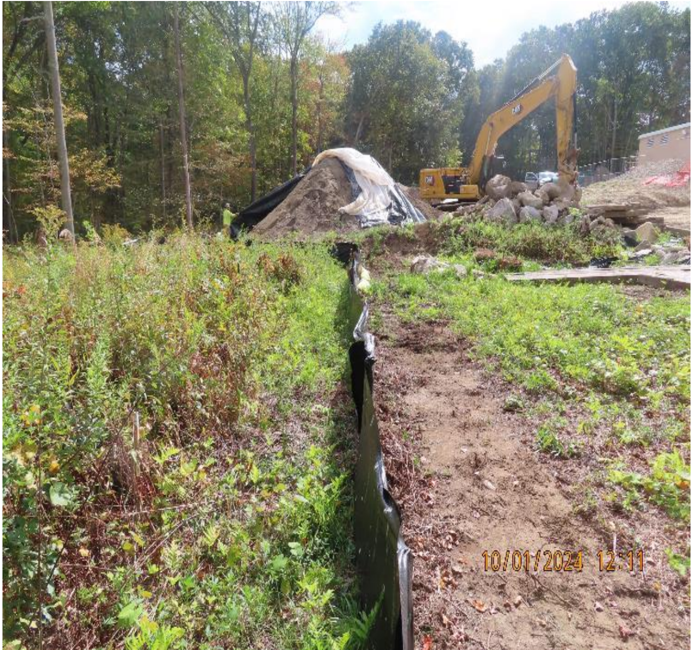
Photo 4: View (looking southeast) at silt fencing along northern site perimeter.
