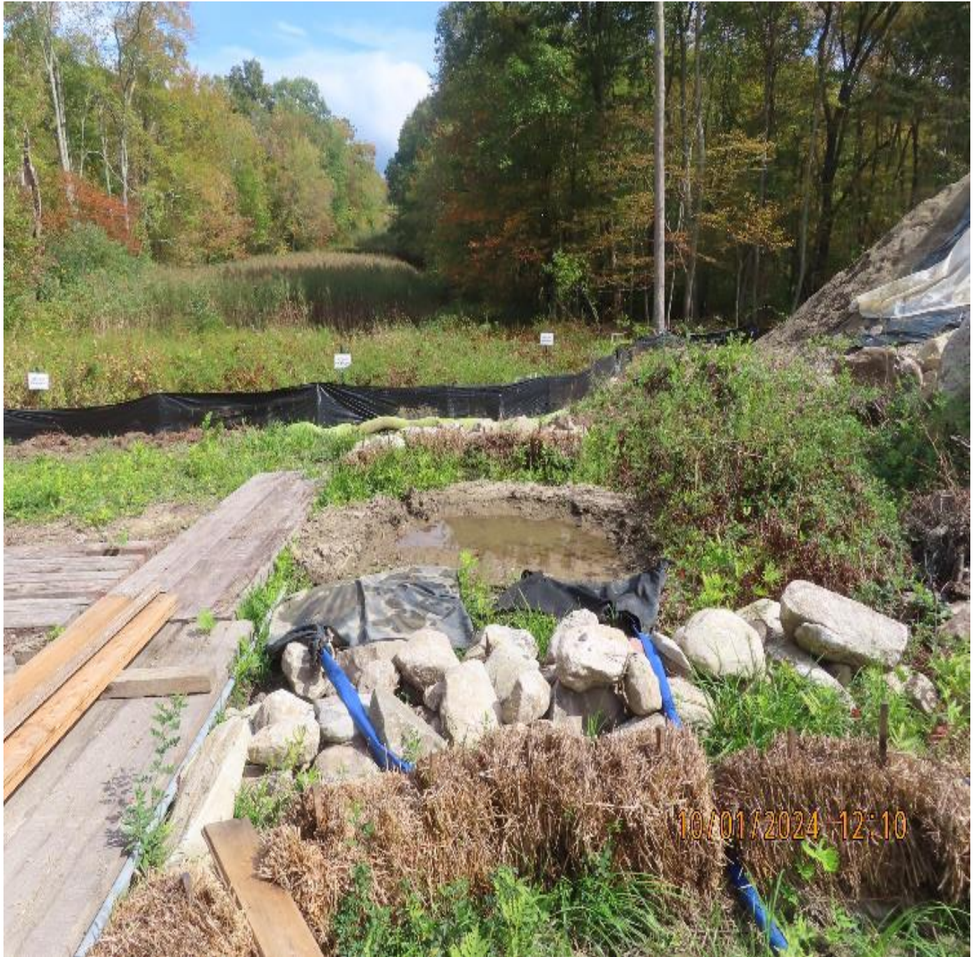
Photo 2: View (looking northeast) at excavation dewatering controls.
