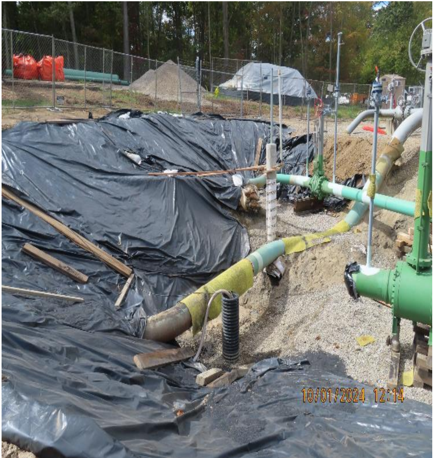
Photo 5: View (looking west) at mechanical work occurring in valve yard.
