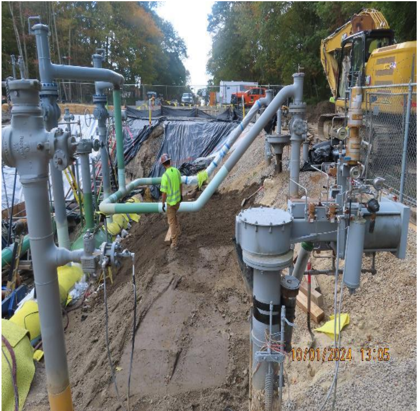
Photo 8: View (looking southwest) at mechanical work in valve yard.
