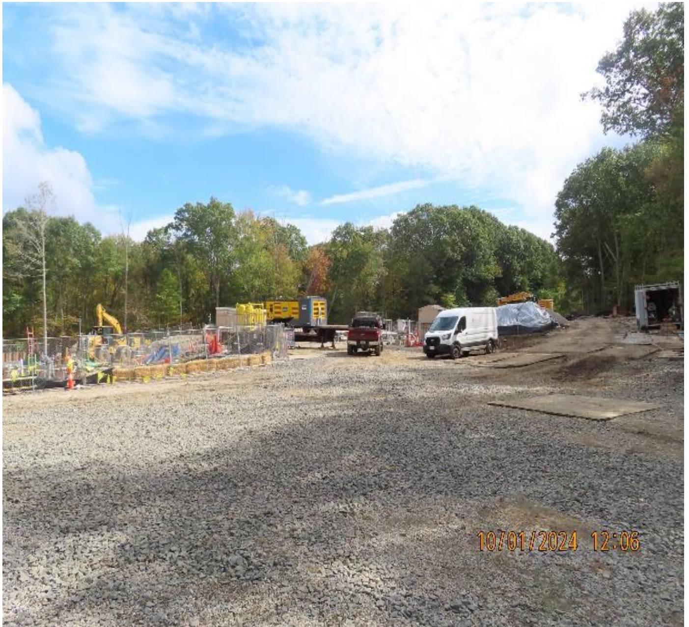
Photo 3: View (looking east) at southern workspace stabilized with stone surfacing.
