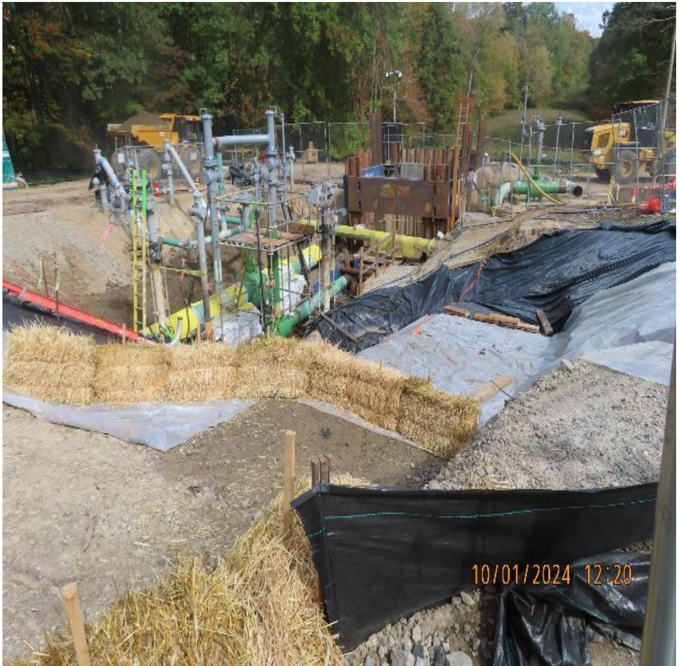
Photo 7: View (looking northwest) at mechanical work occurring in valve yard.
