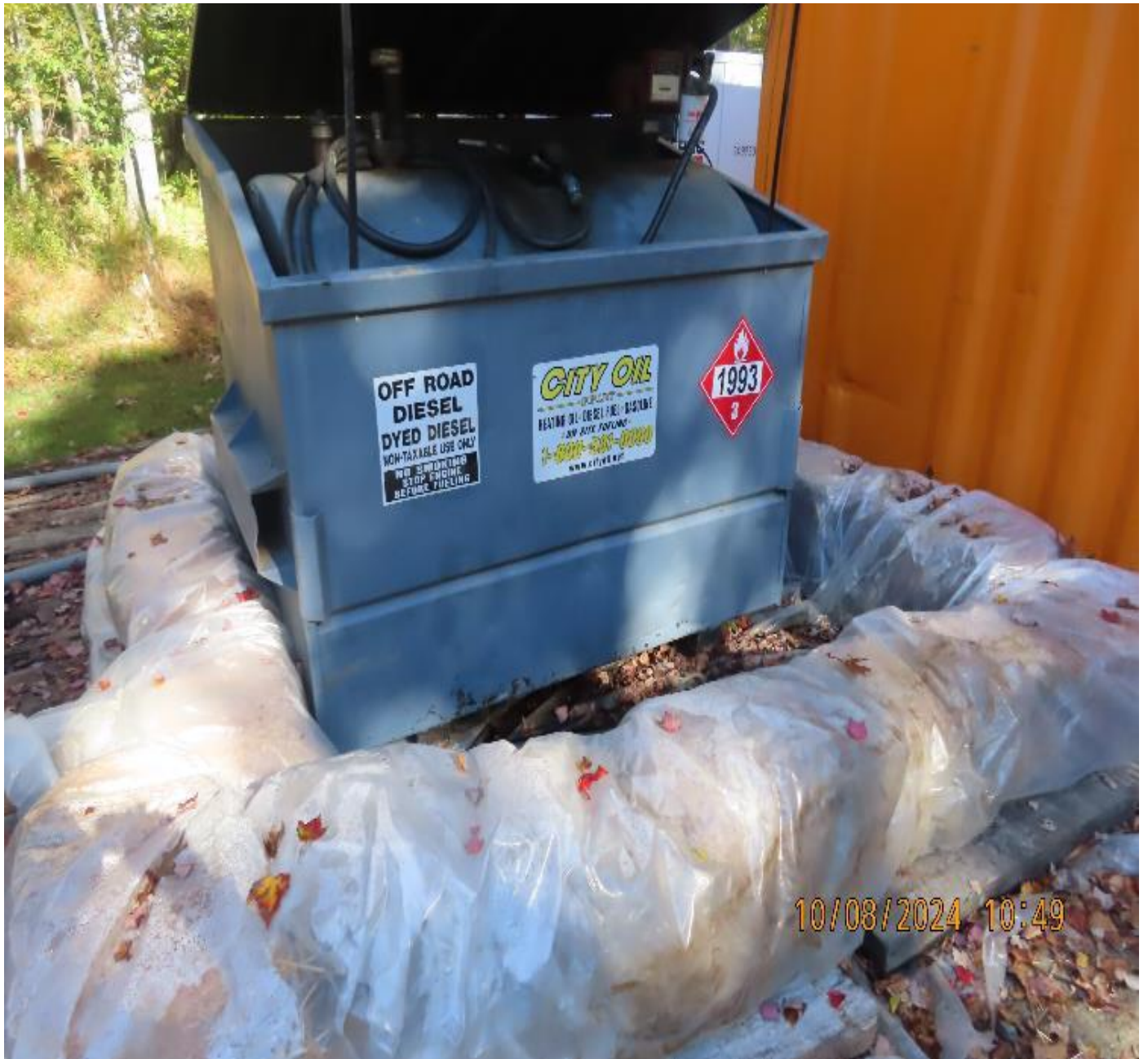
Photo 7: View (looking northwest) of containment around fuel tank.
