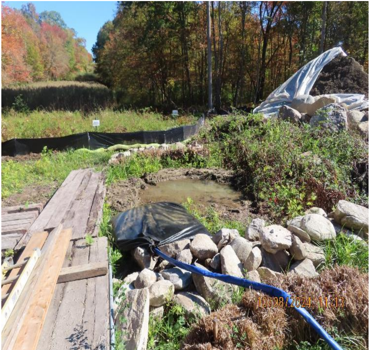
Photo 3: View (looking northeast) of excavation dewatering discharge controls.
