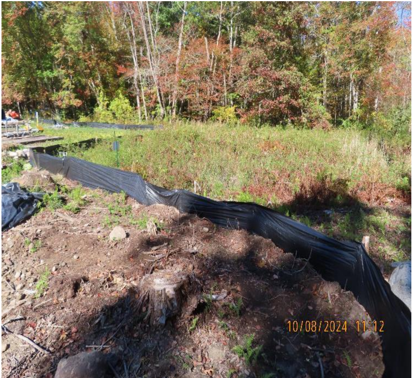
Photo 5: View (looking northwest) of silt fence near wetland W-CZ-01.
