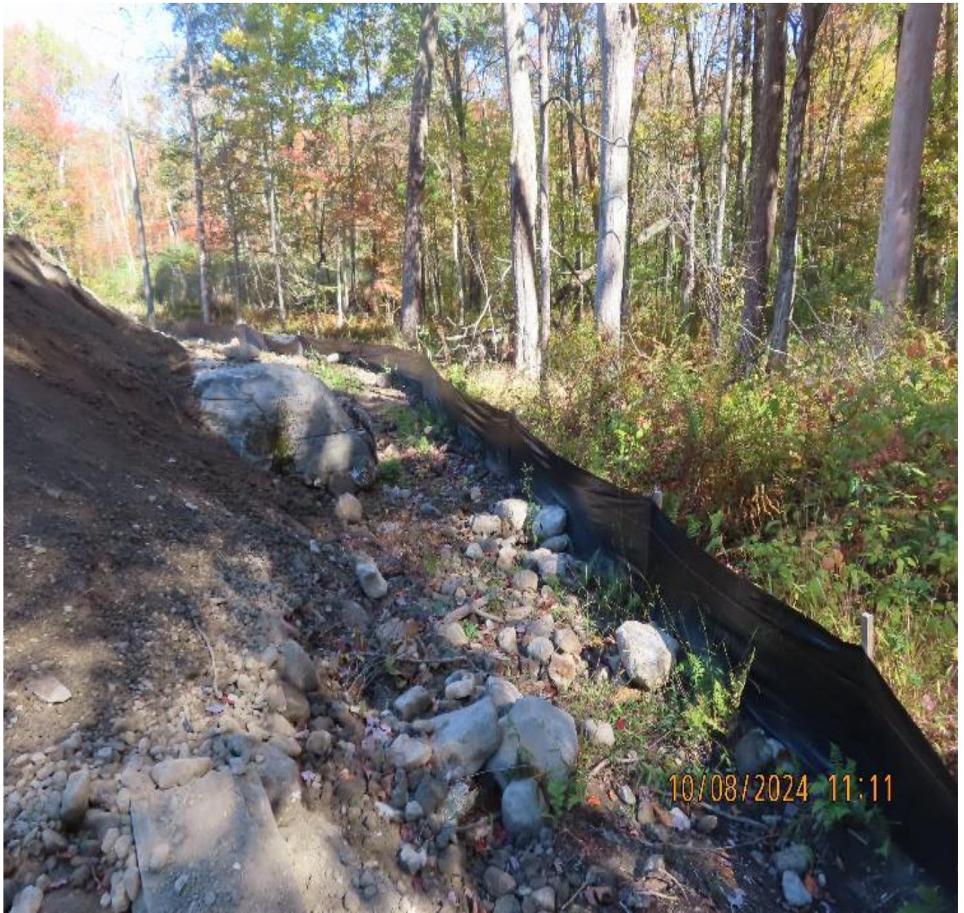
Photo 4: View (looking north) of silt fence downslope of excavated soil stockpile.
