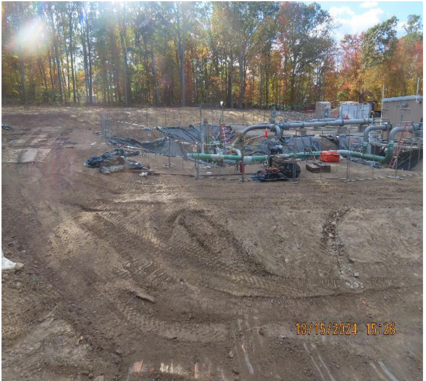
Photo 5: View (looking southwest) of E-System 30-inch tie-in excavation area after backfilling.
