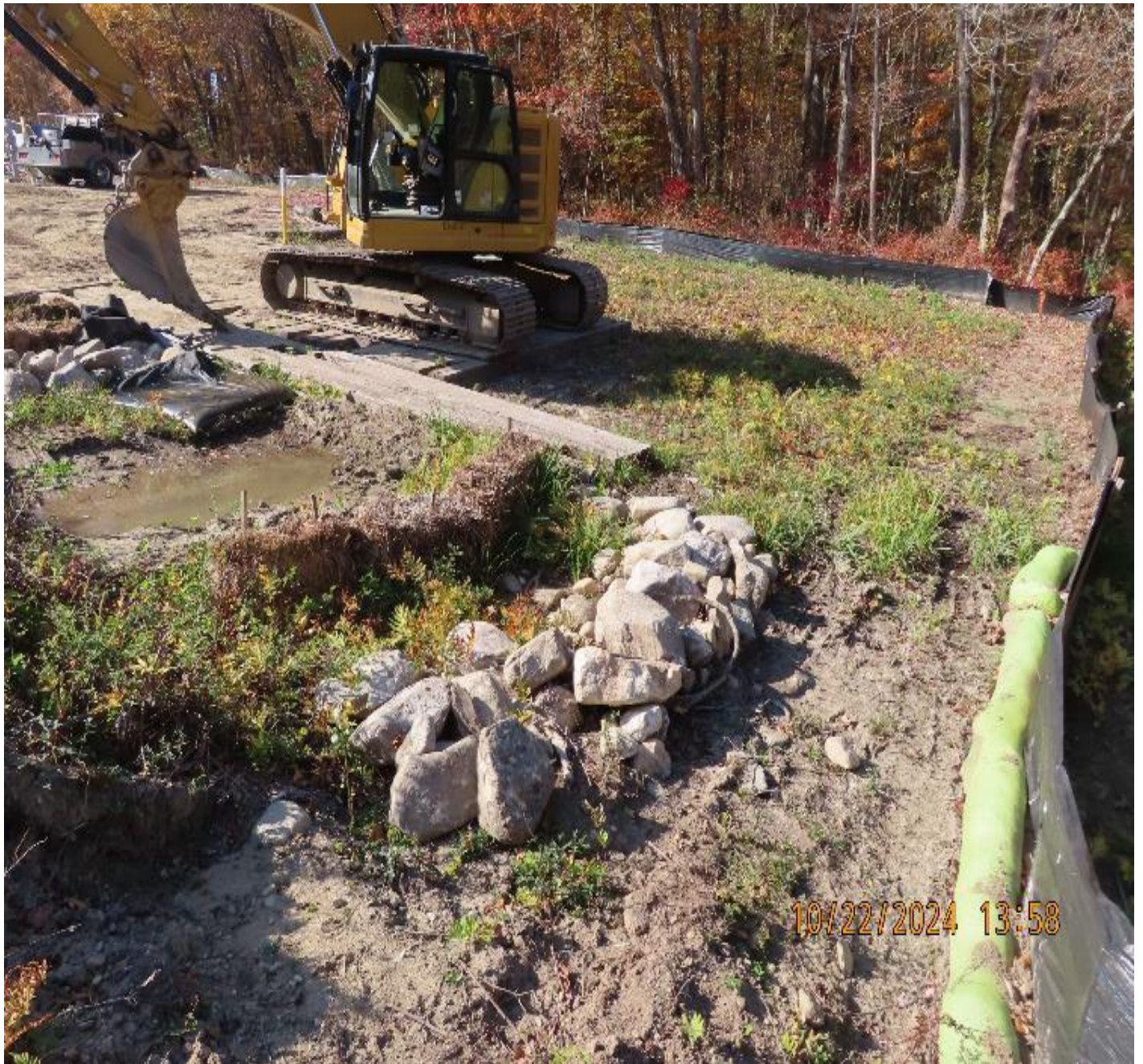
Photo 6: View (looking west) of excavation dewatering discharge area will full ground infiltration.
