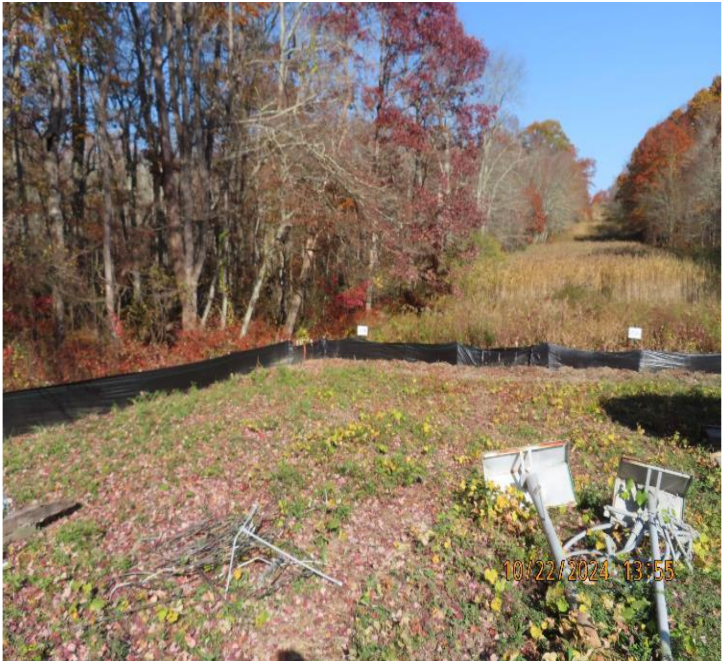
Photo 8: View (looking north) of perimeter ECDs and vegetative buffer protection for wetland W-CZ-01.
