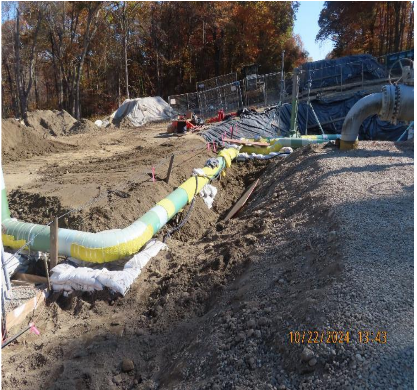
Photo 5: View (looking southeast) of partial backfilling completes along 16-inch outlet piping.
