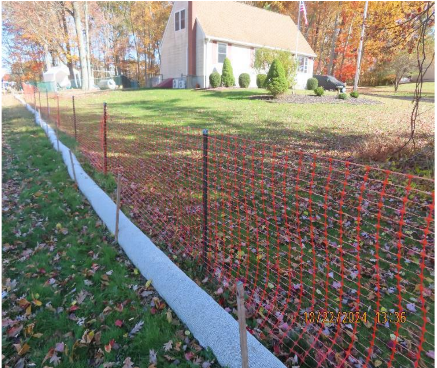
Photo 1: View (looking northeast) of perimeter ECDs and security fencing along the east side of site access.
