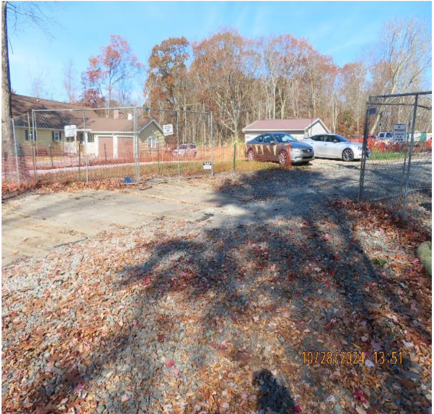
Photo 1: View (looking northwest) of work site entrance off Hop River Road.
