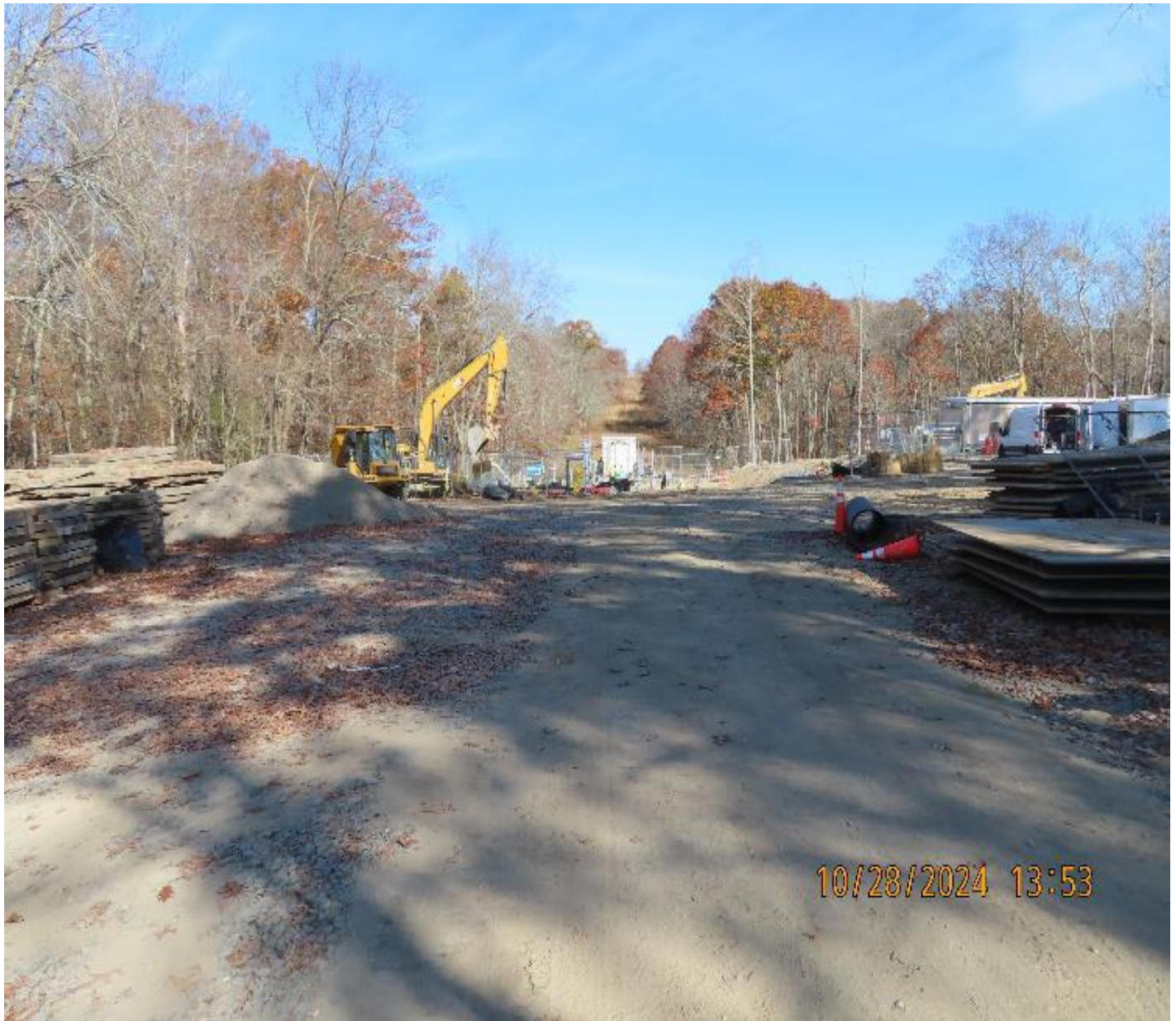
Photo 2: View (looking northeast) of approach to the valve yard work area.
