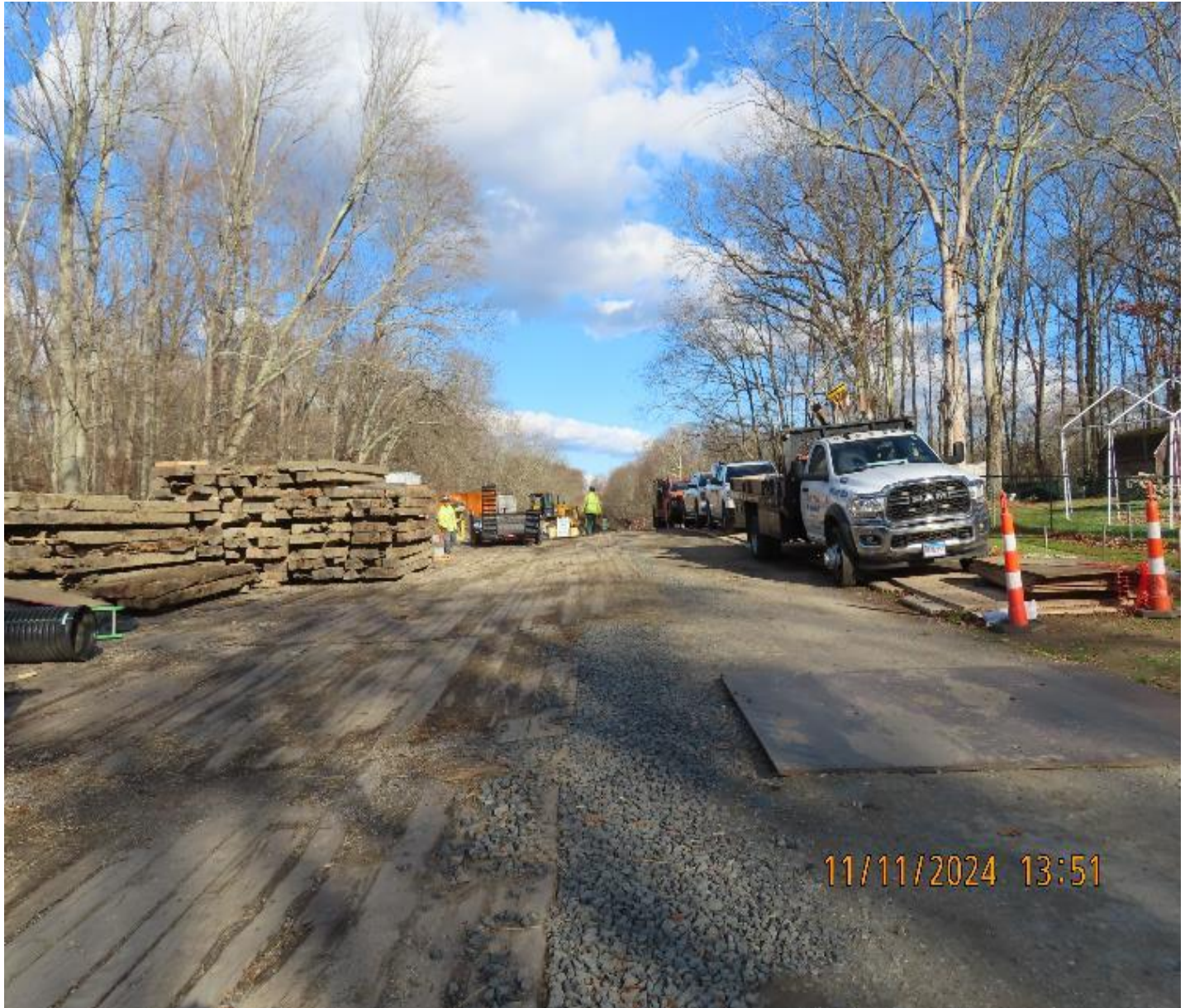
Photo 1: View (looking northeast) of staging area.
