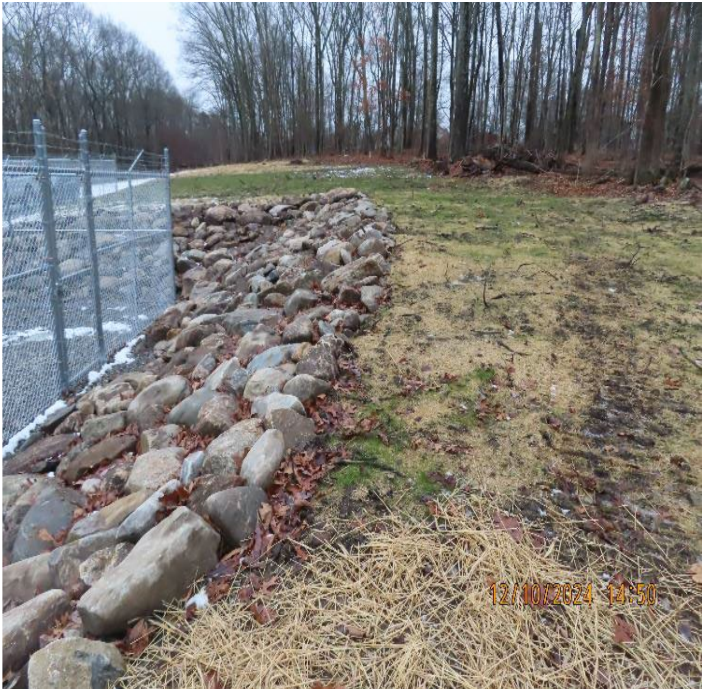
Photo 4: View (looking southeast) of conditions behind the new RTU building.
