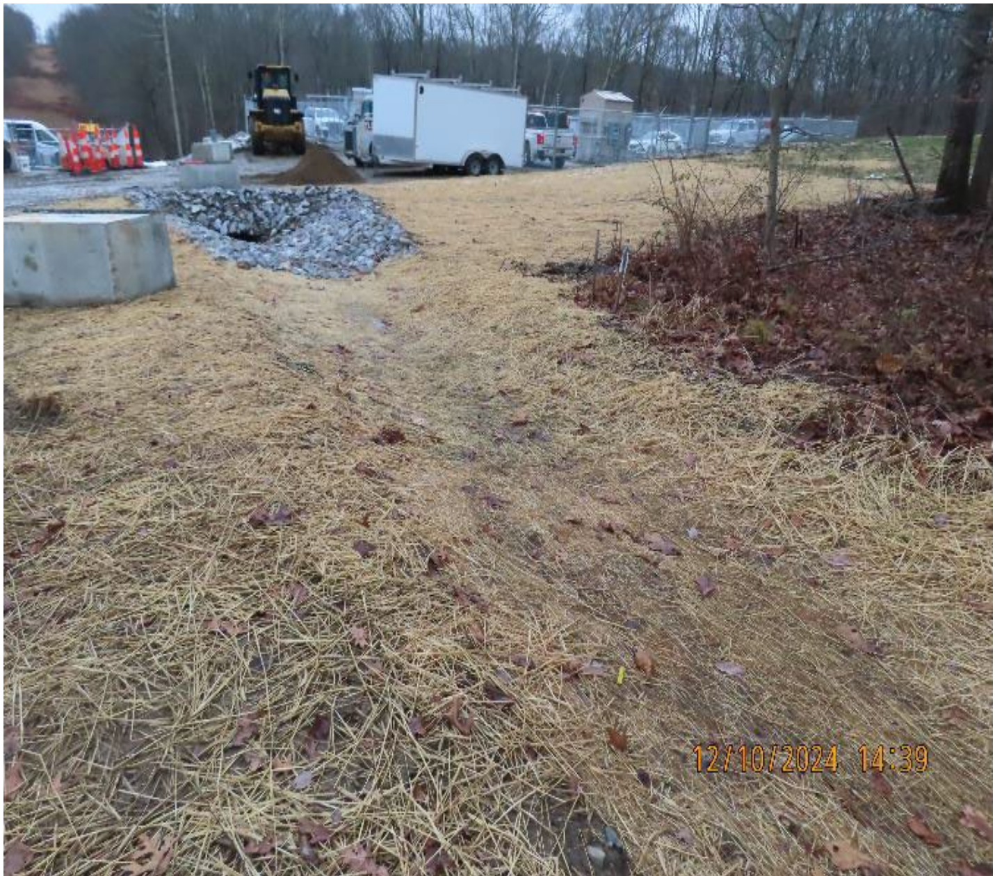
Photo 1: View (looking northeast) of stormwater drainage swale upgradient of culvert inlet.
