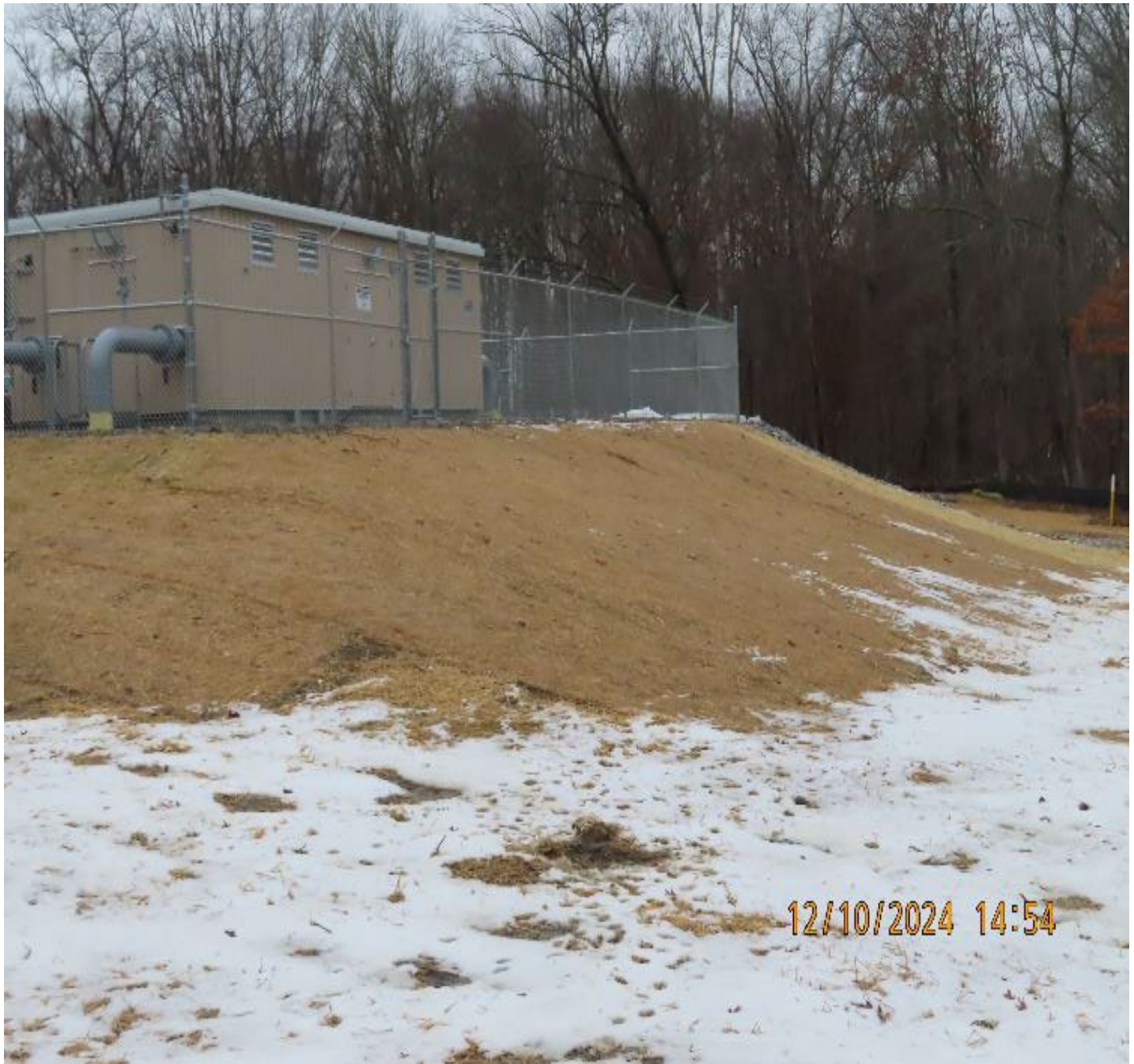
Photo 6: View (looking west) of stabilized embankment north of the new regulator building.
