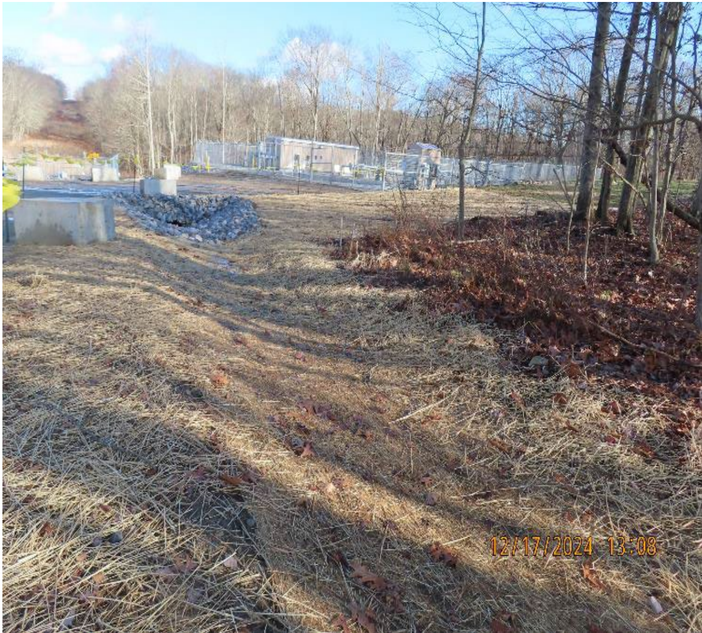
Photo 4: View (looking northeast) of drainage swale draining to culvert in central area of site.
