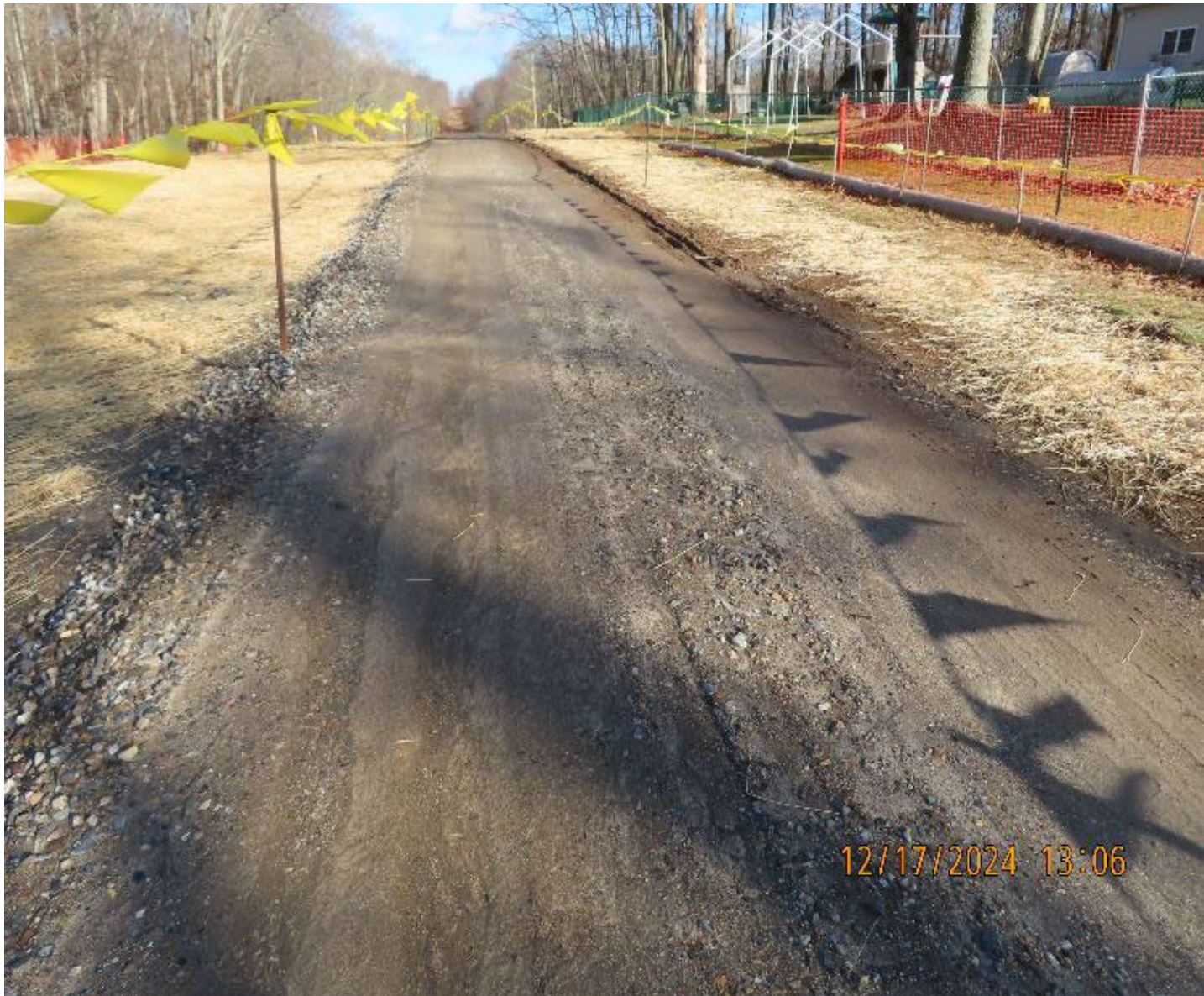
Photo 2: View (looking northeast) off access road after contractor demobilization.
