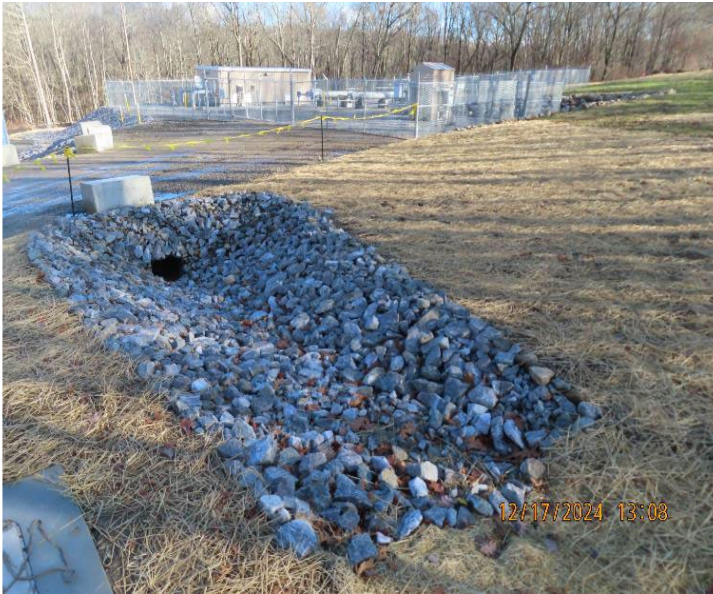
Photo 5: View (looking east) of rock-stabilized culvert inlet.
