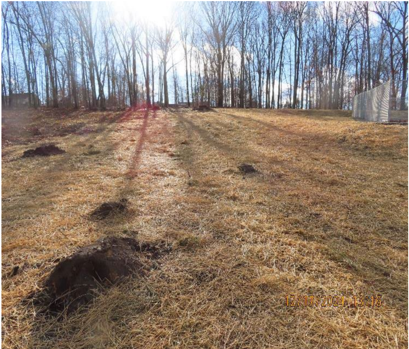
Photo 10: View (looking southeast) of stabilized area on east side of new regulator building.
