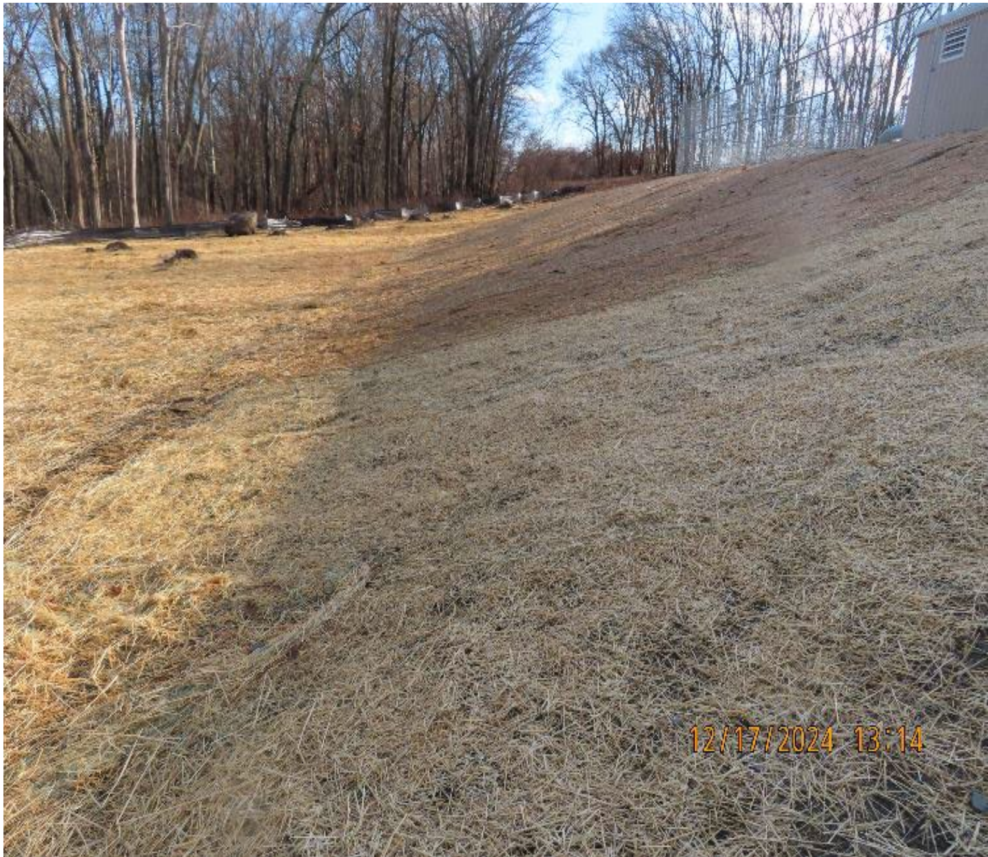
Photo 9: View (looking east) of stabilized slope along north side of the new regulator building.
