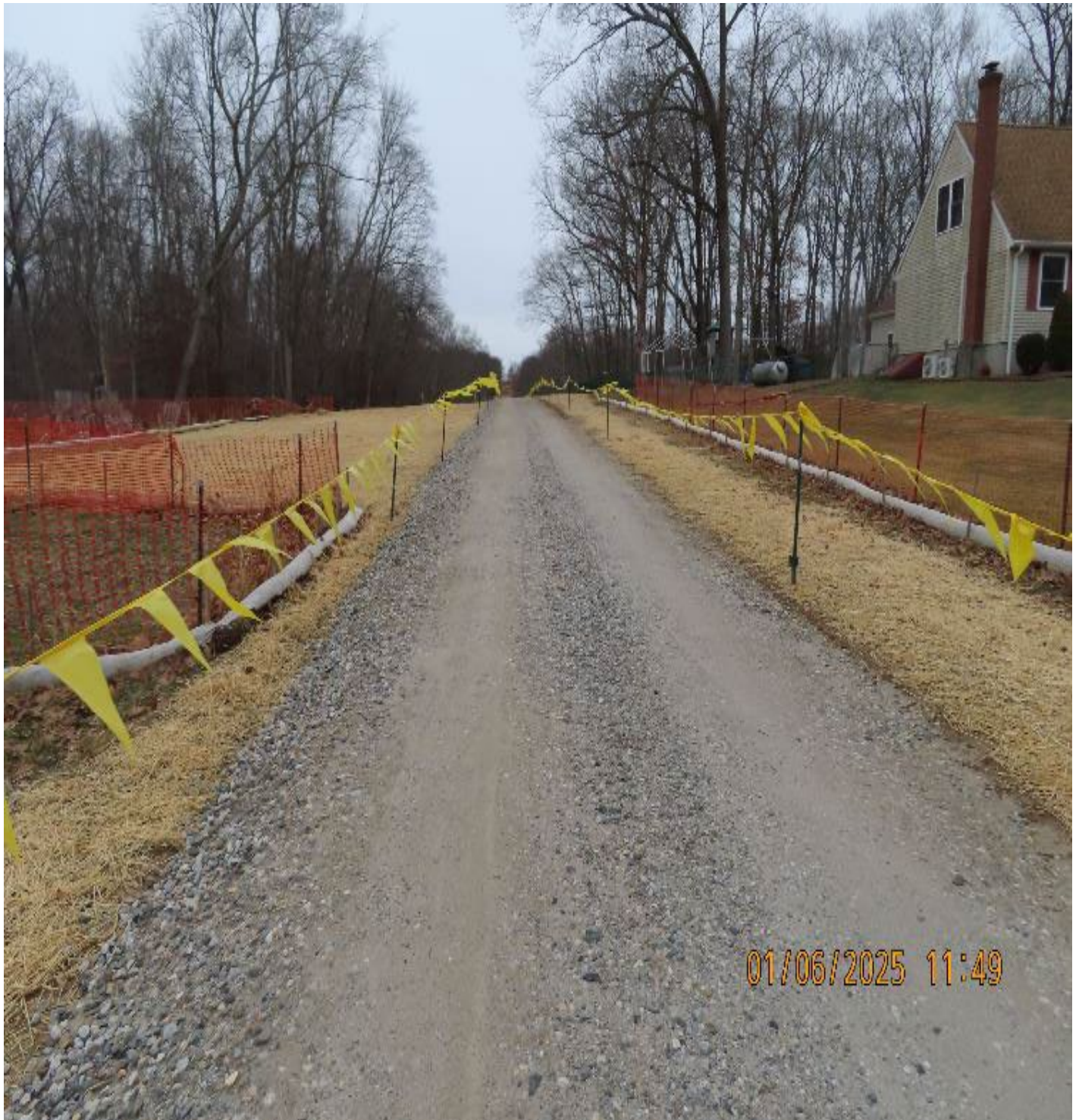
Photo 2: View (looking northeast) of access road conditions in residential area.
