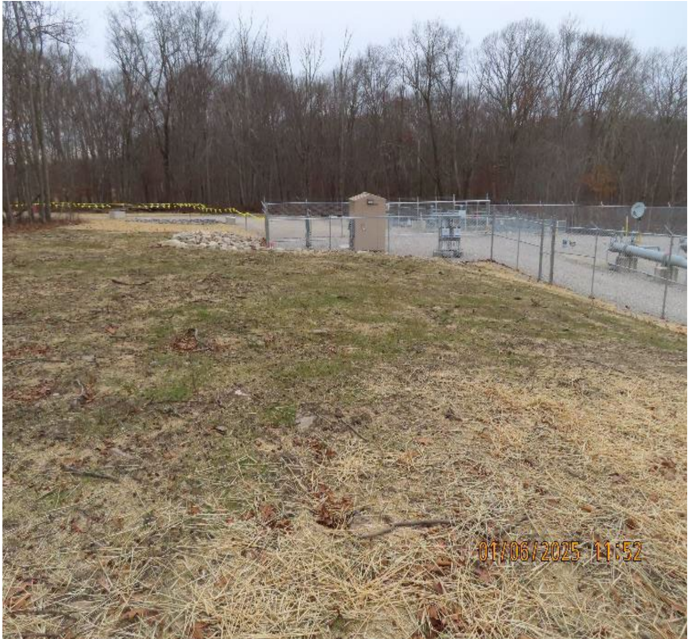
Photo 5: View (looking northwest) of south workspace near valve station.
