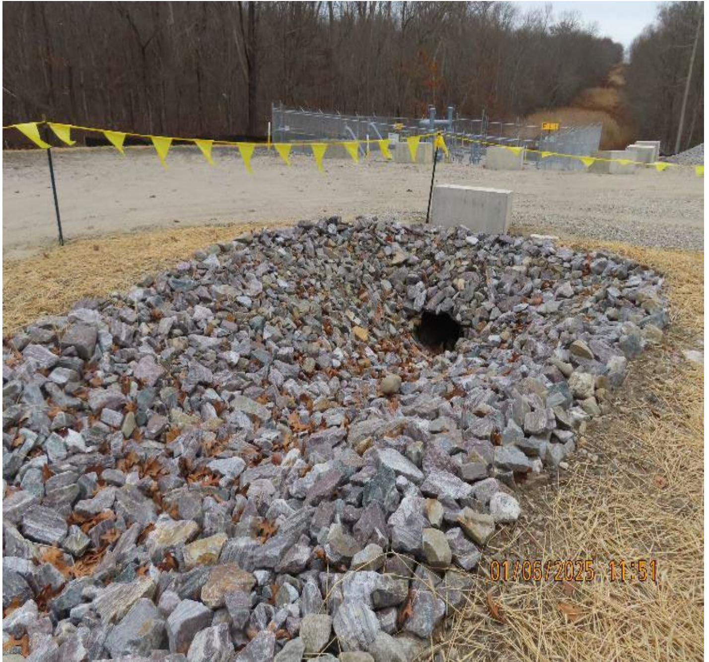
Photo 4: View (looking north) of access road culverted drainage crossing.
