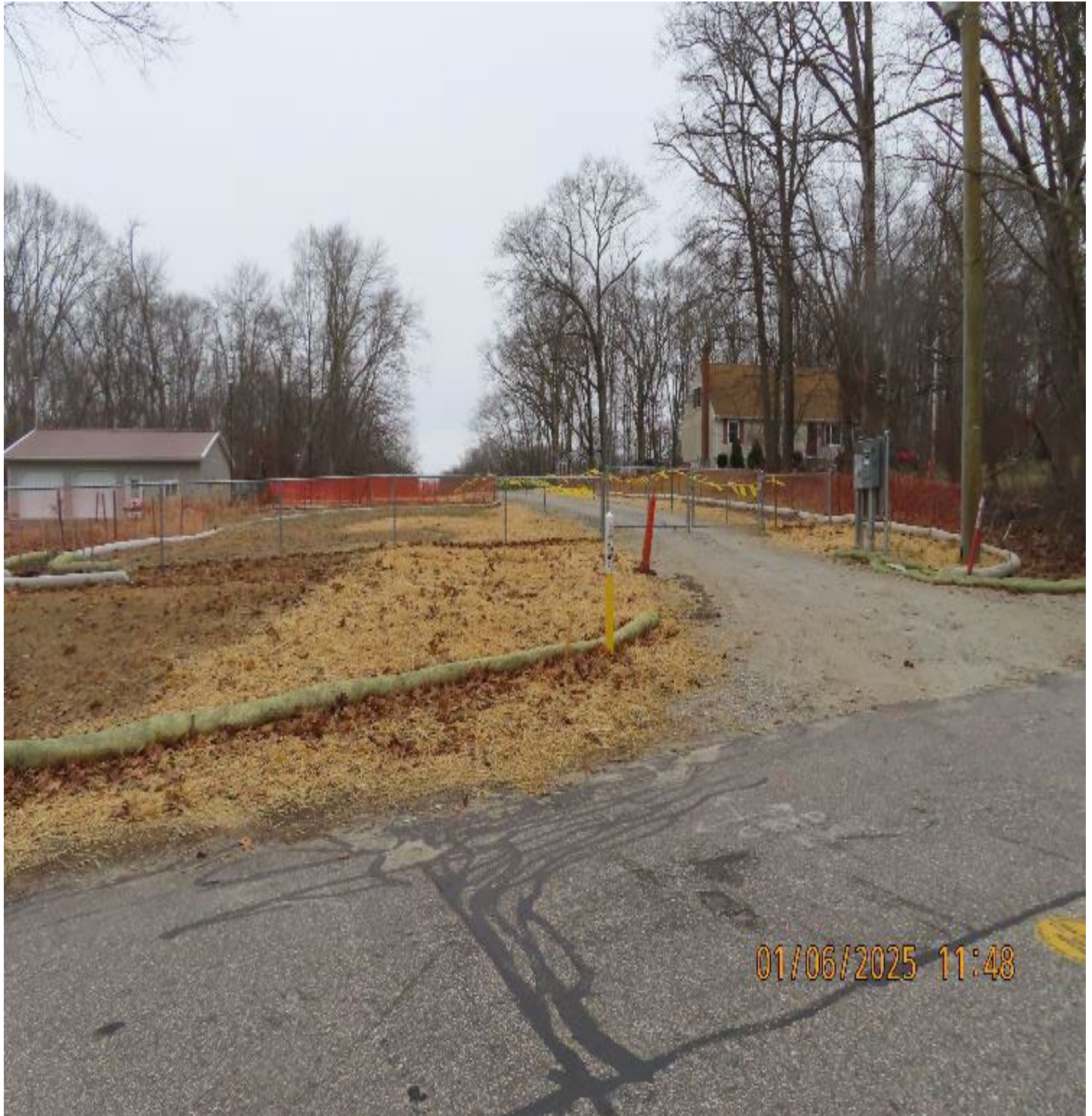
Photo 1: View (looking northeast) of site entrance off Hop River Road.
