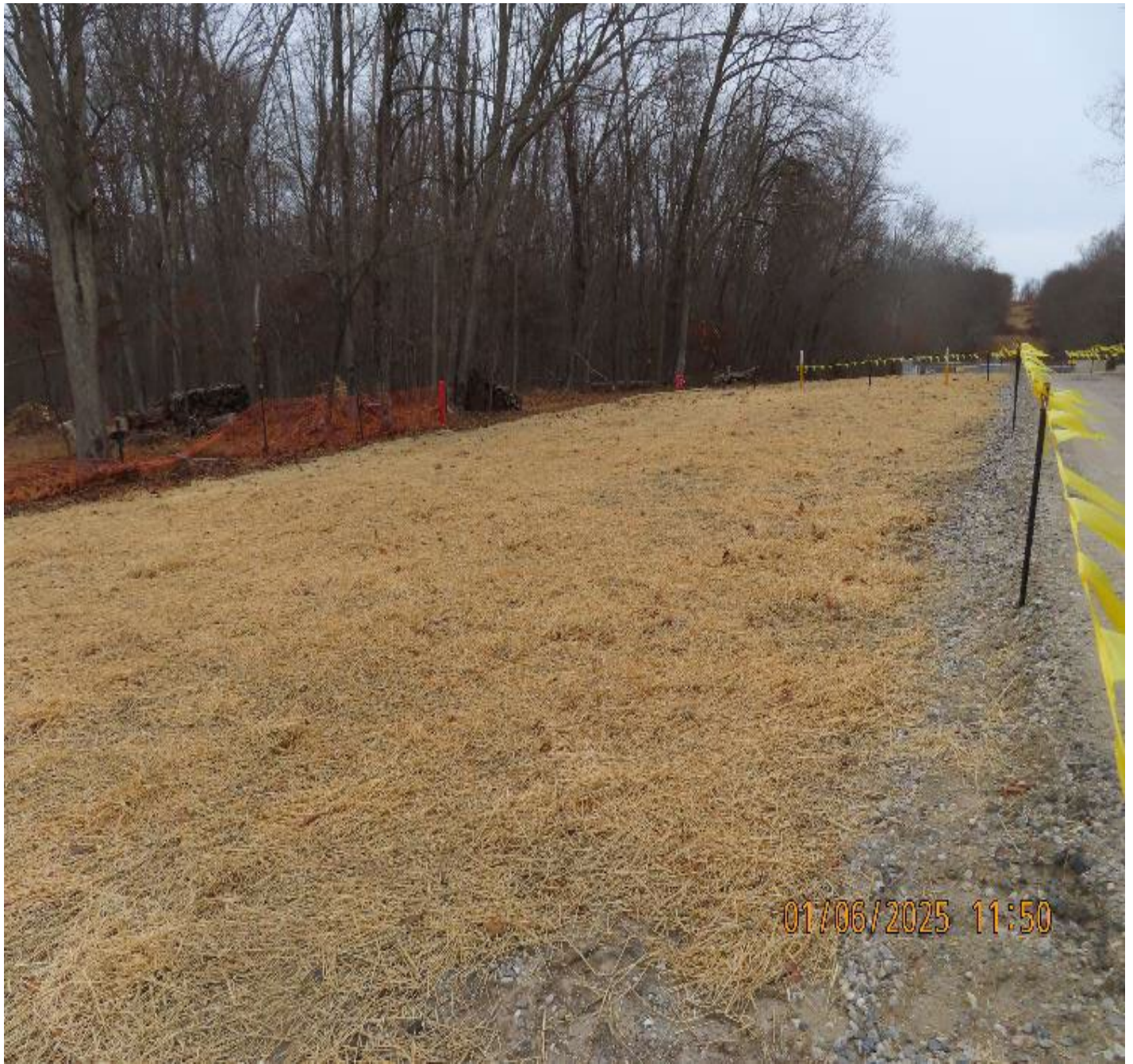
Photo 3: View (looking northeast) of former job trailer and refueling area.
