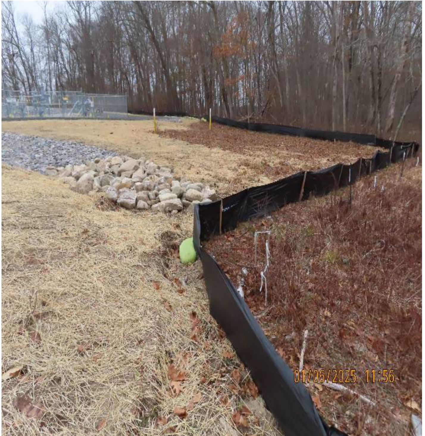
Photo 7: View (looking west) at silt fencing along wetland W-CZ-01.
