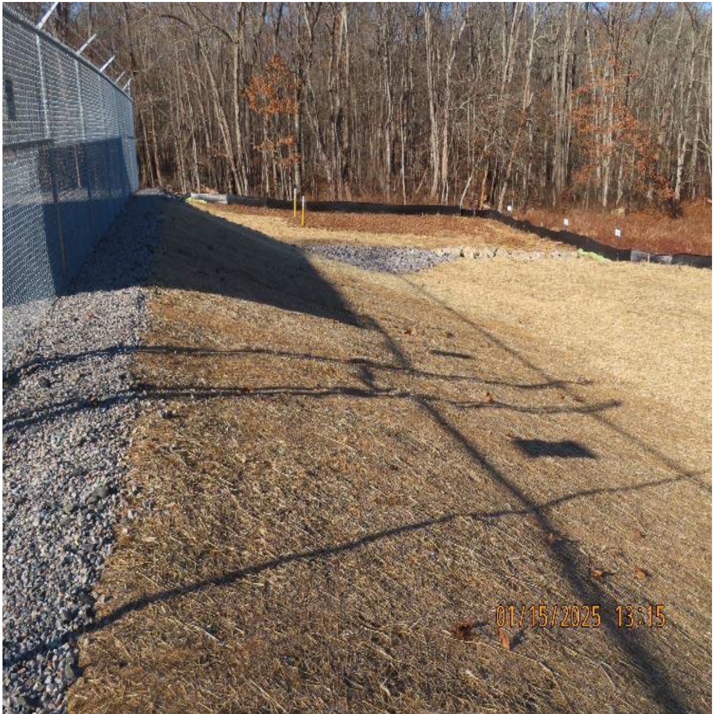
Photo 7: View (looking northwest) of north embankment for the new regulatory building.
