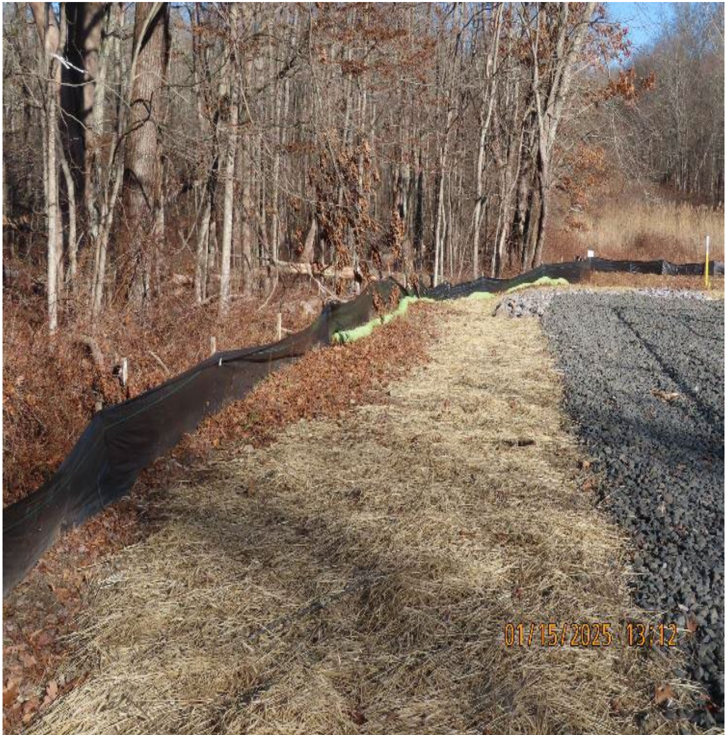
Photo 5: View (looking northeast) of silt fence and filter sock along western workspace boundary.
