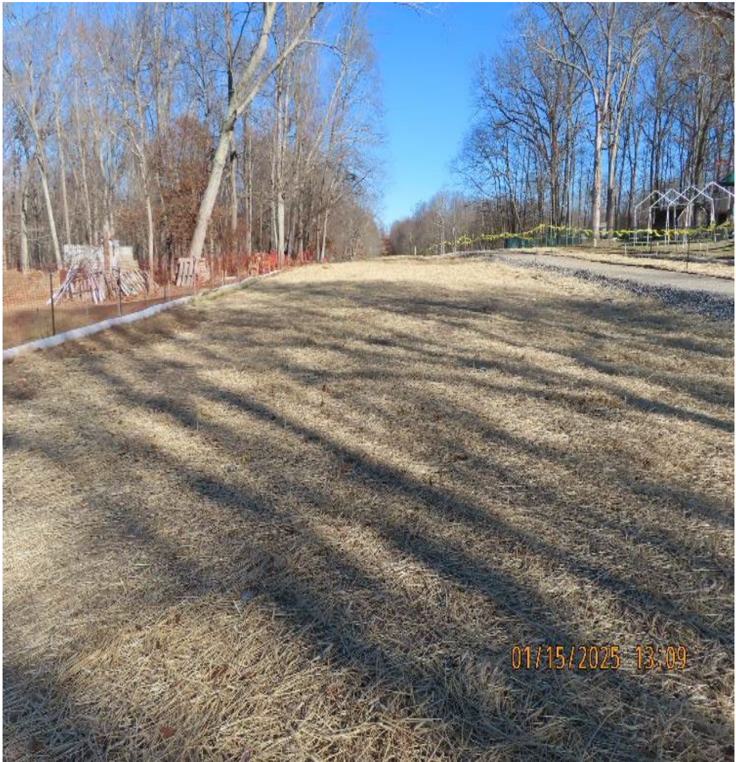
Photo 2: View (looking northeast) of former staging area south of main construction area.
