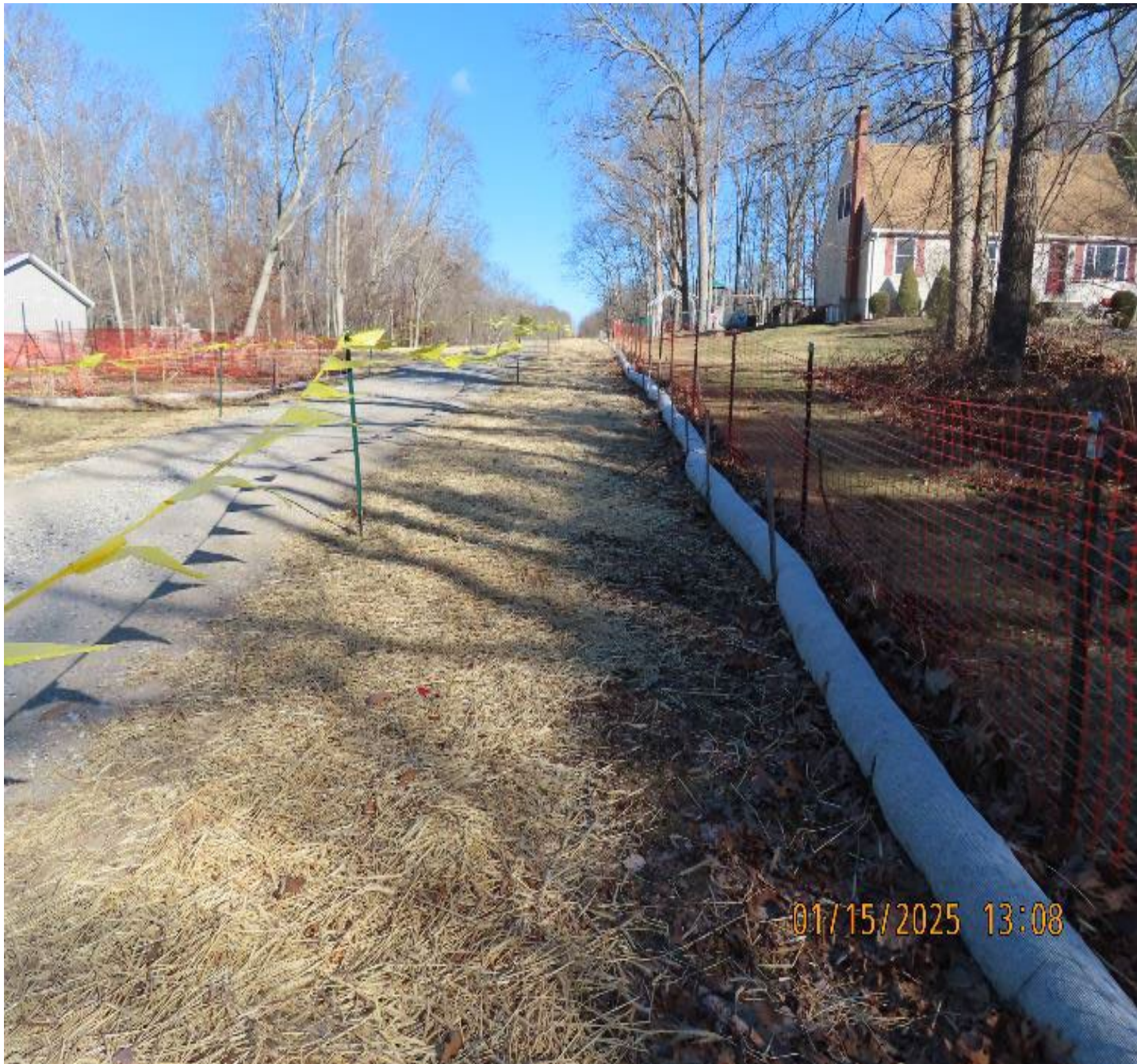
Photo 1: View (looking northeast) of access from Hop River Road.
