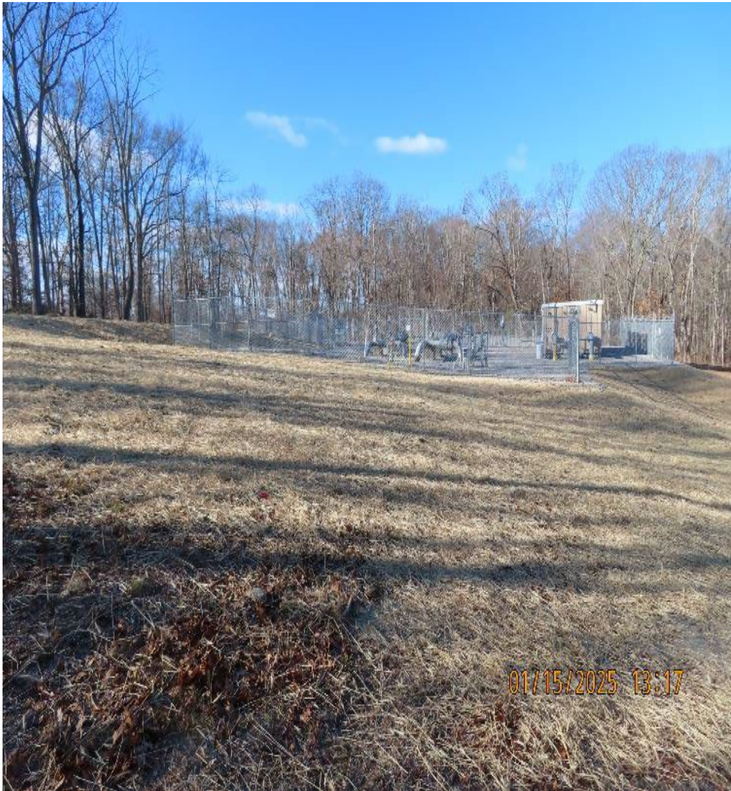
Photo 8: View (looking northwest) of stabilized conditions around the valve yard.
