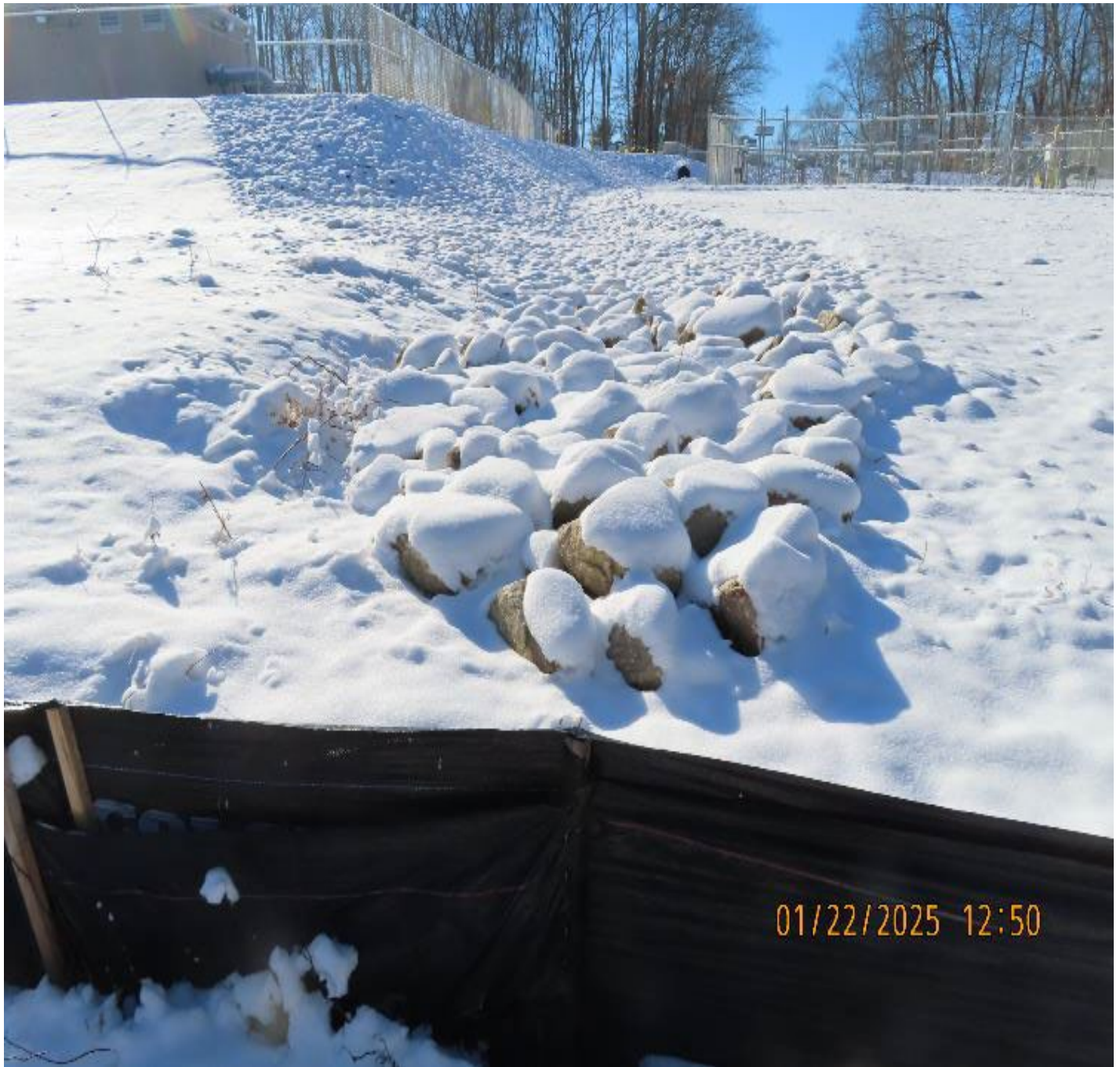
Photo 3: View (looking south) of culvert outlet and rock-armored drainage swale.
