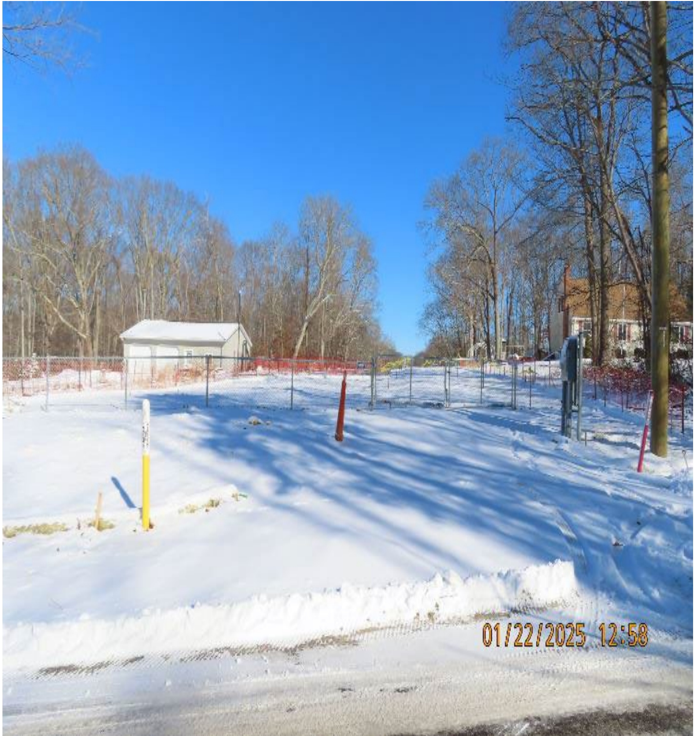
Photo 1: View (looking northeast) of site entrance off Hop River Road.
