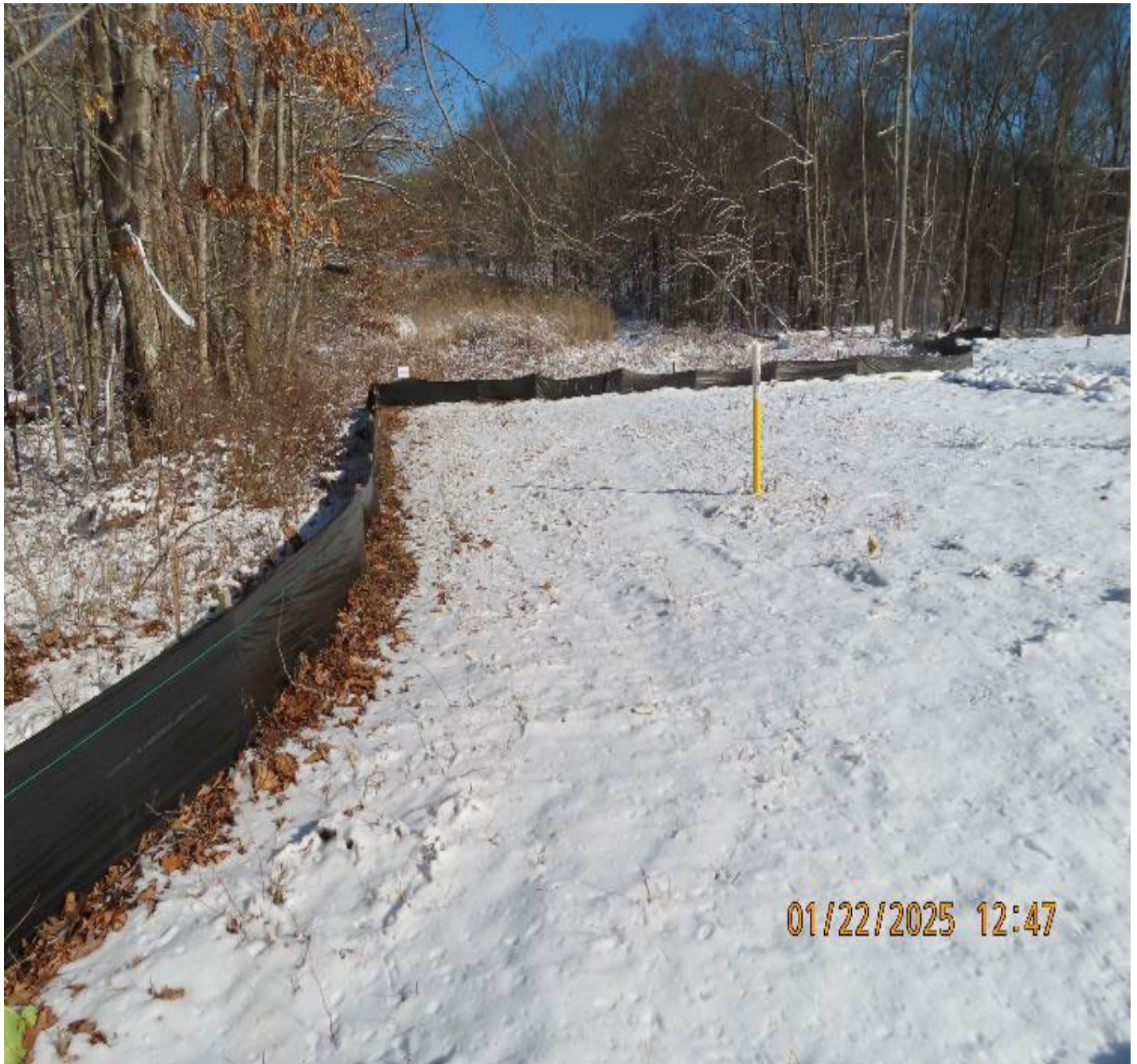
Photo 5: View (looking northeast) of silt fence along northwest corner of former workspace.
