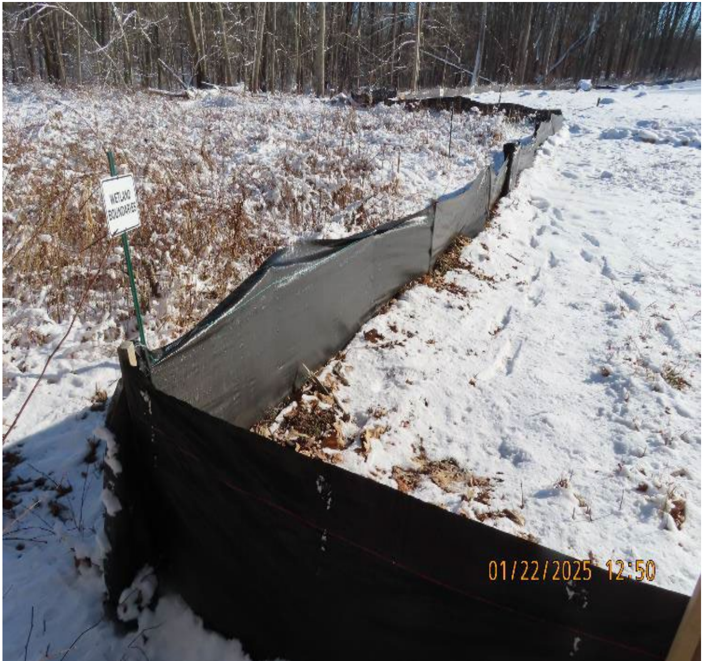
Photo 6: View (looking southeast) of silt fencing along Wetland W-CZ-01.
