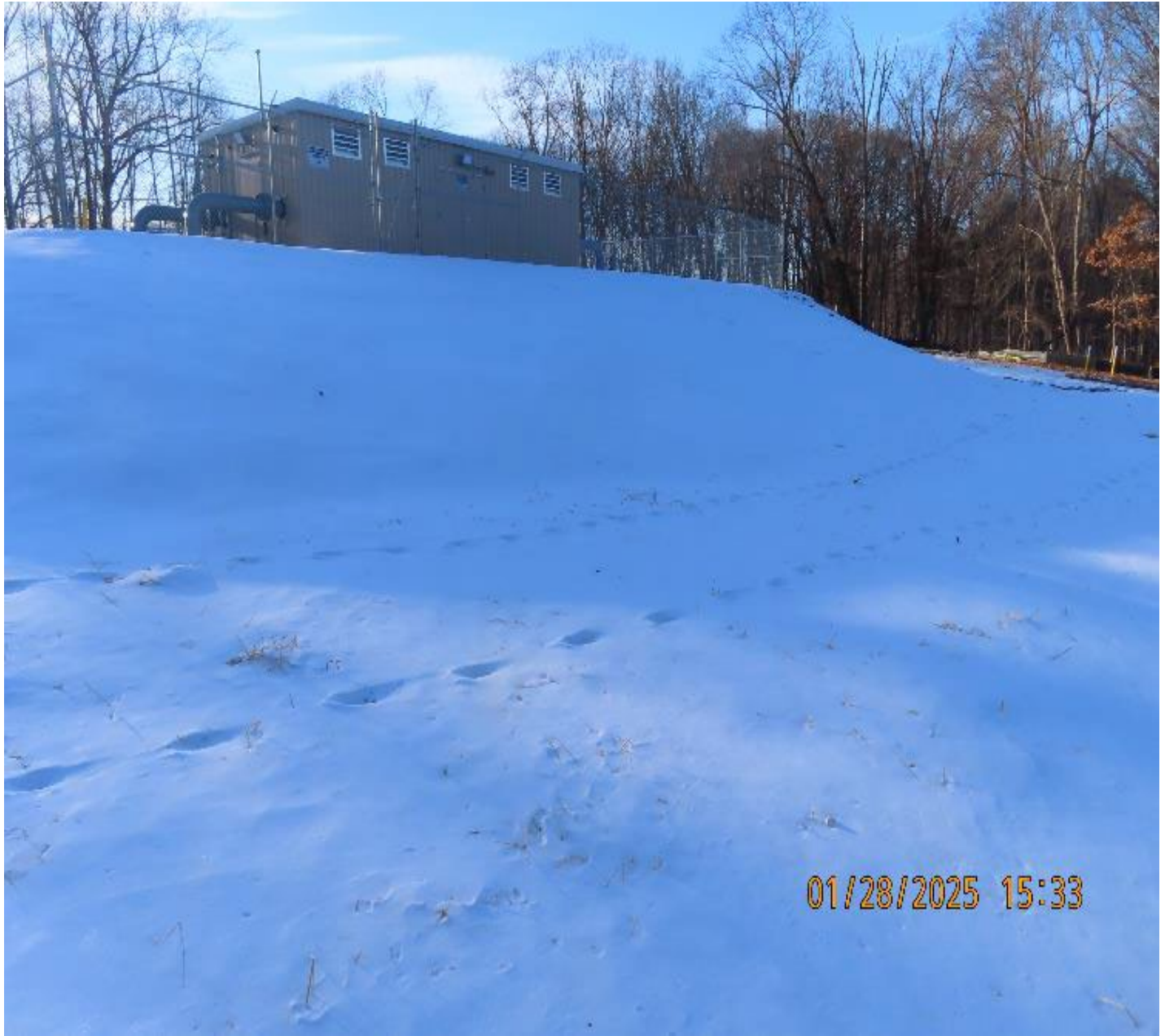
Photo 4: View (looking west) of new regulator building.
