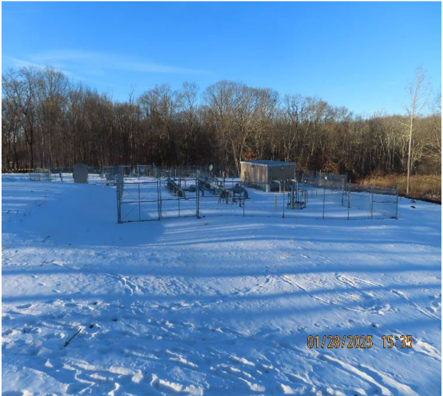
Photo 3: View (looking north) of valve yard.
