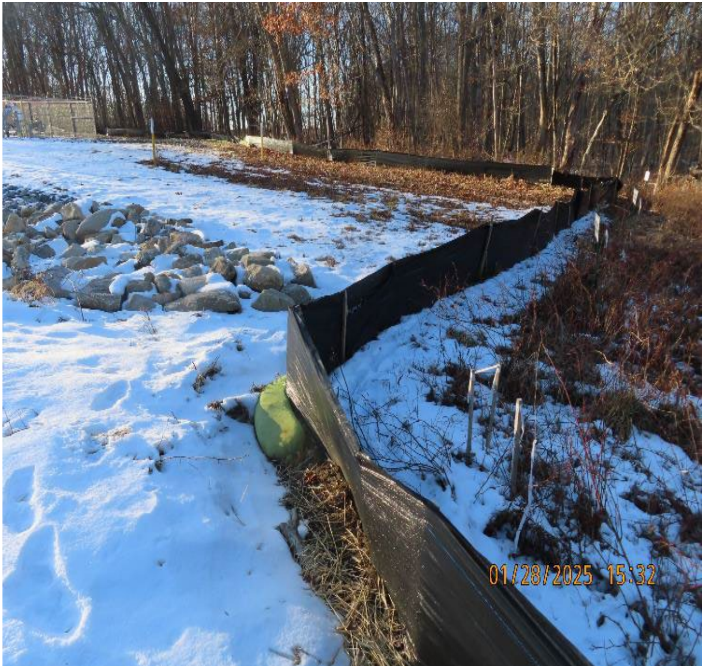
Photo 6: View (looking west) of erosion controls along wetland W-CZ-01.
