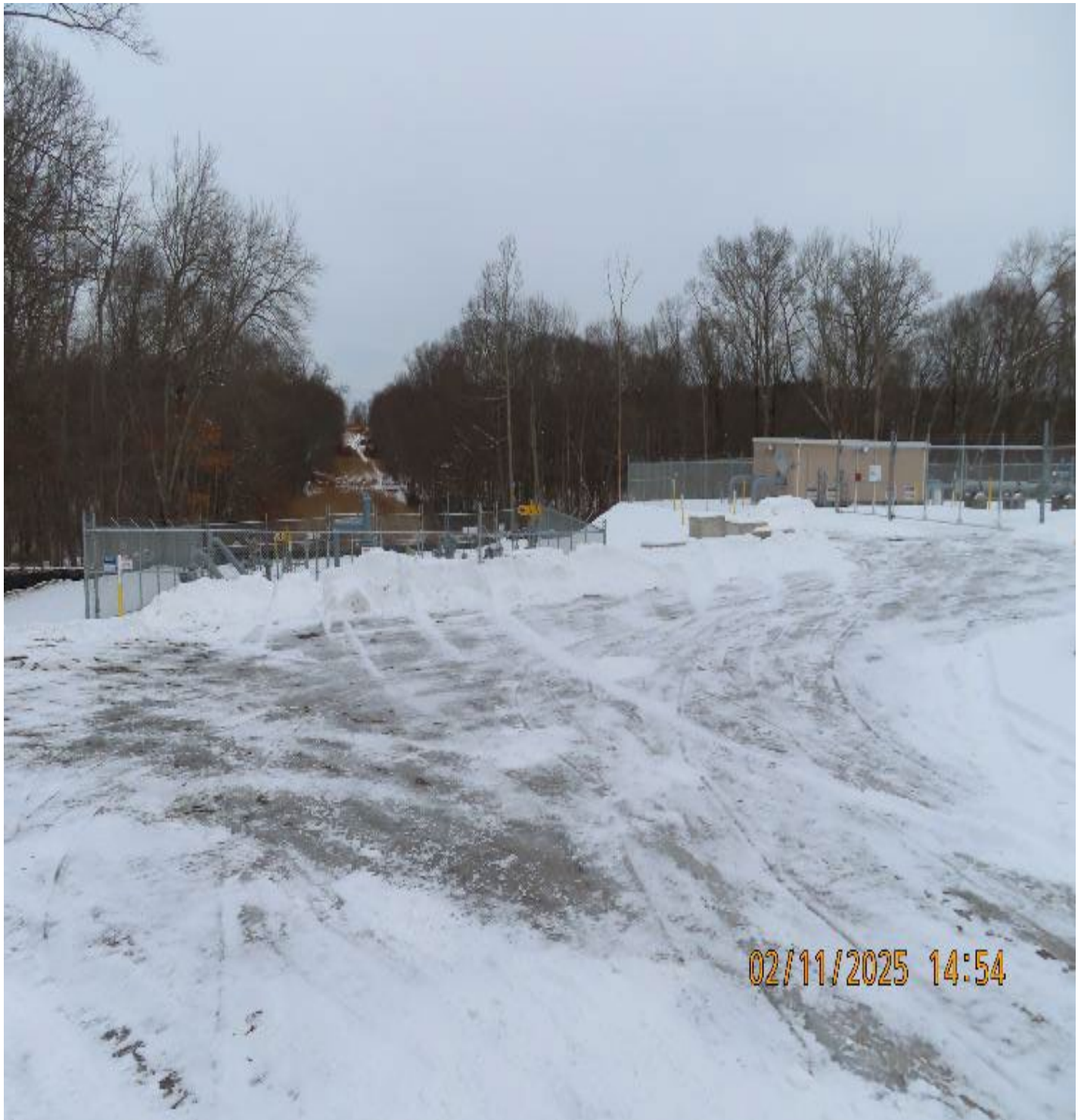
Photo 2: View (looking northeast) of plowed access road to valve yard.
