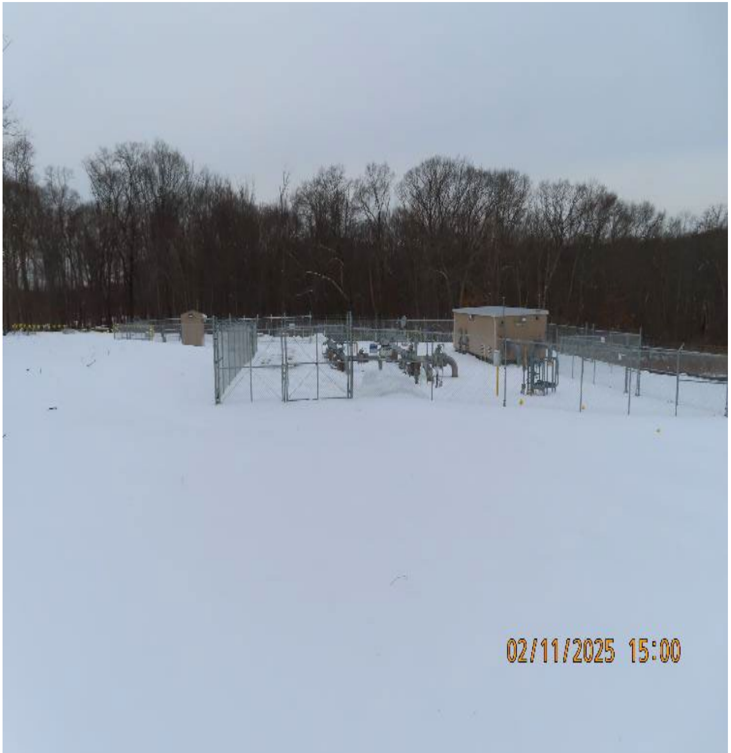
Photo 5: View (looking northwest) at snow covered conditions around valve yard.
