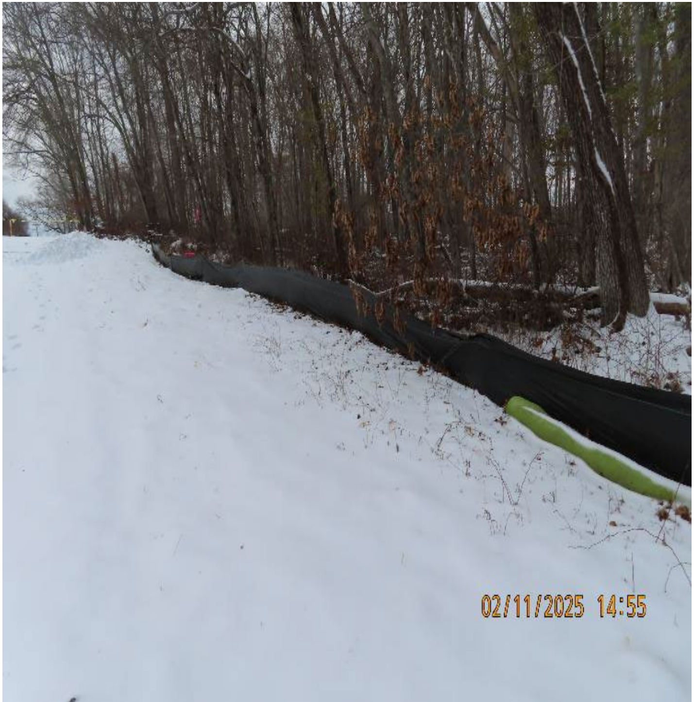
Photo 3: View (looking southwest) of silt fence along west workspace boundary.
