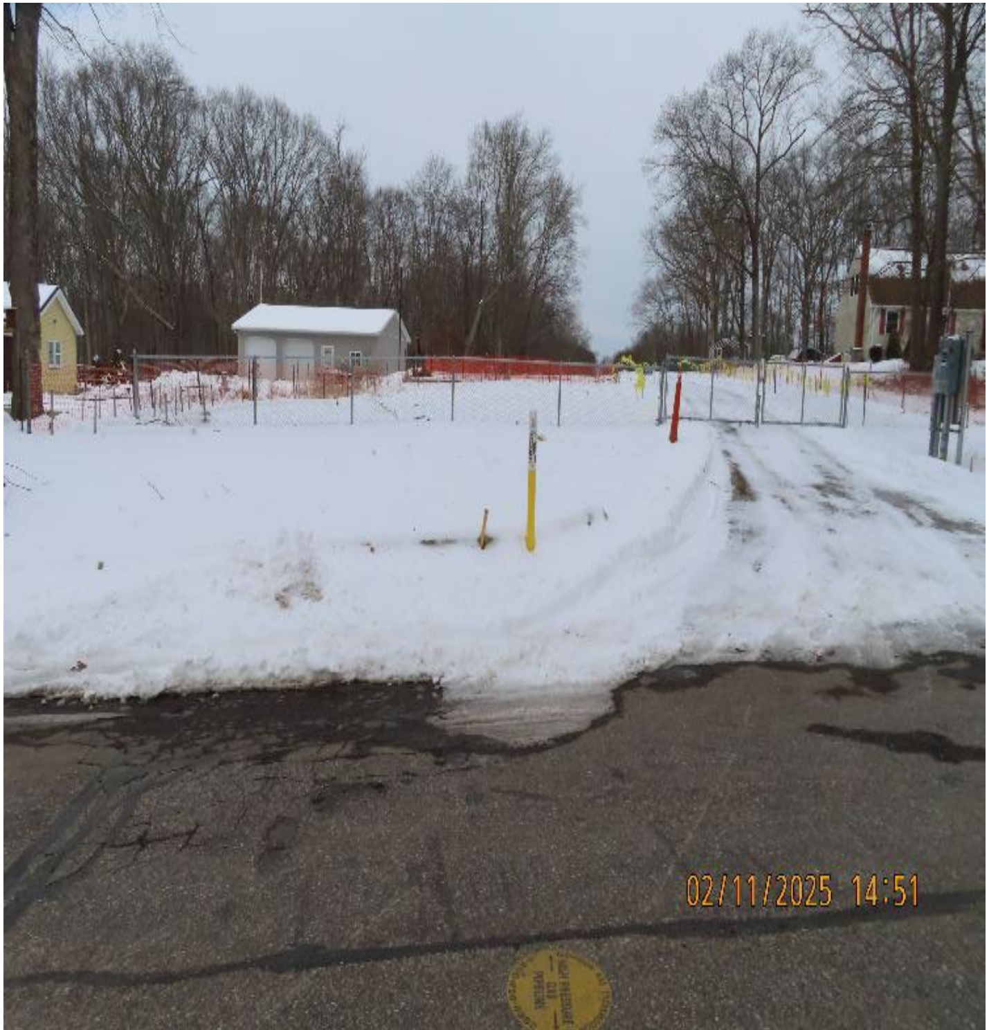
Photo 1: View (looking northeast) of site access from Hop River Road.
