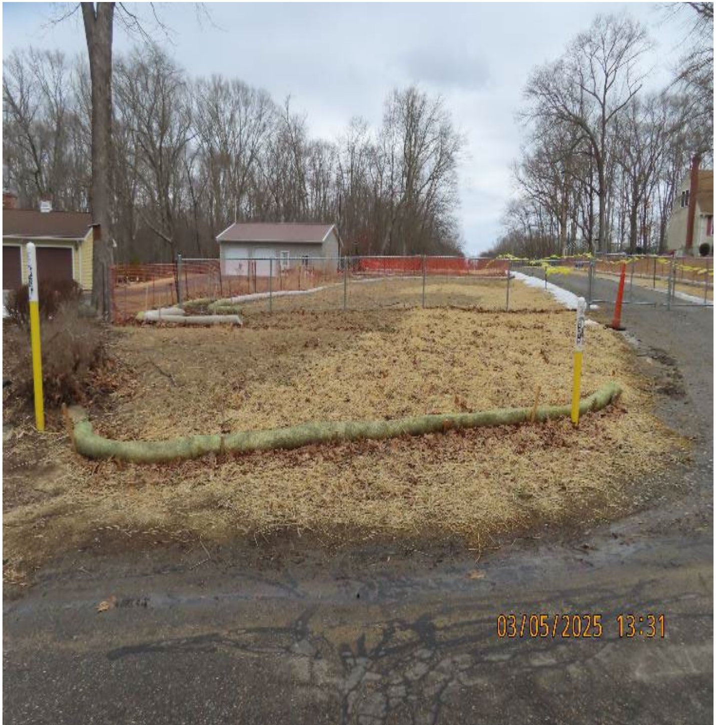
Photo 1: View (looking northeast) of site entrance from Hop River Road.
