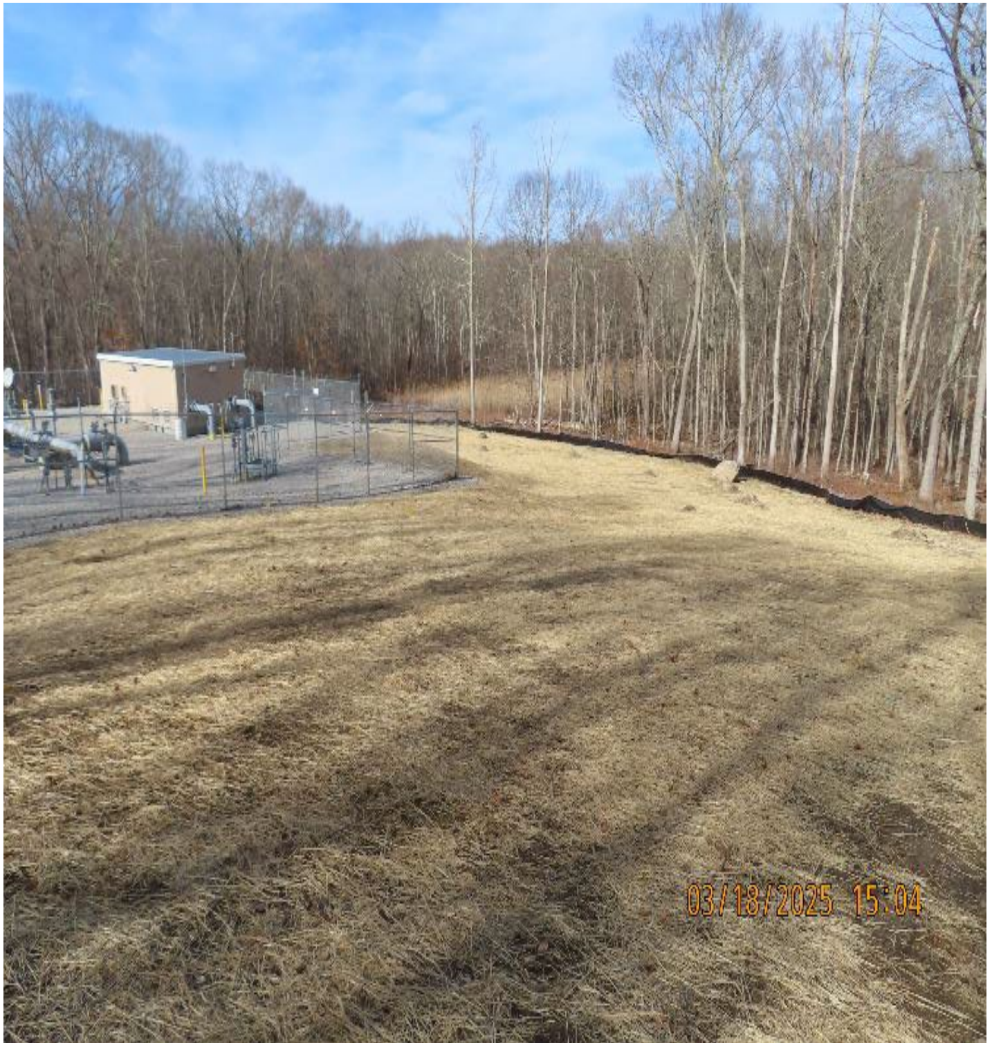
Photo 5: View (looking north) of stabilized areas around the valve yard and new regulator building.
