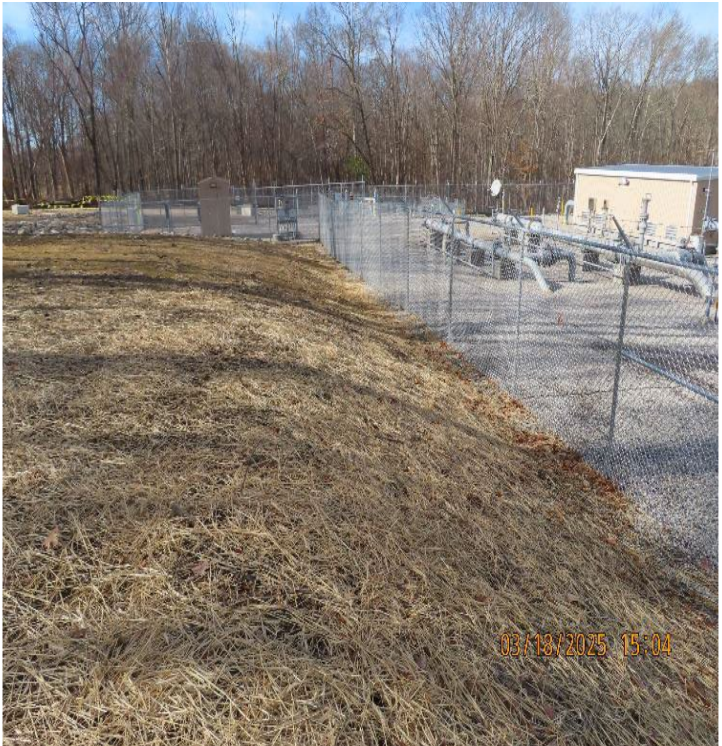
Photo 4: View (looking west) of stabilized slope south of the valve yard.
