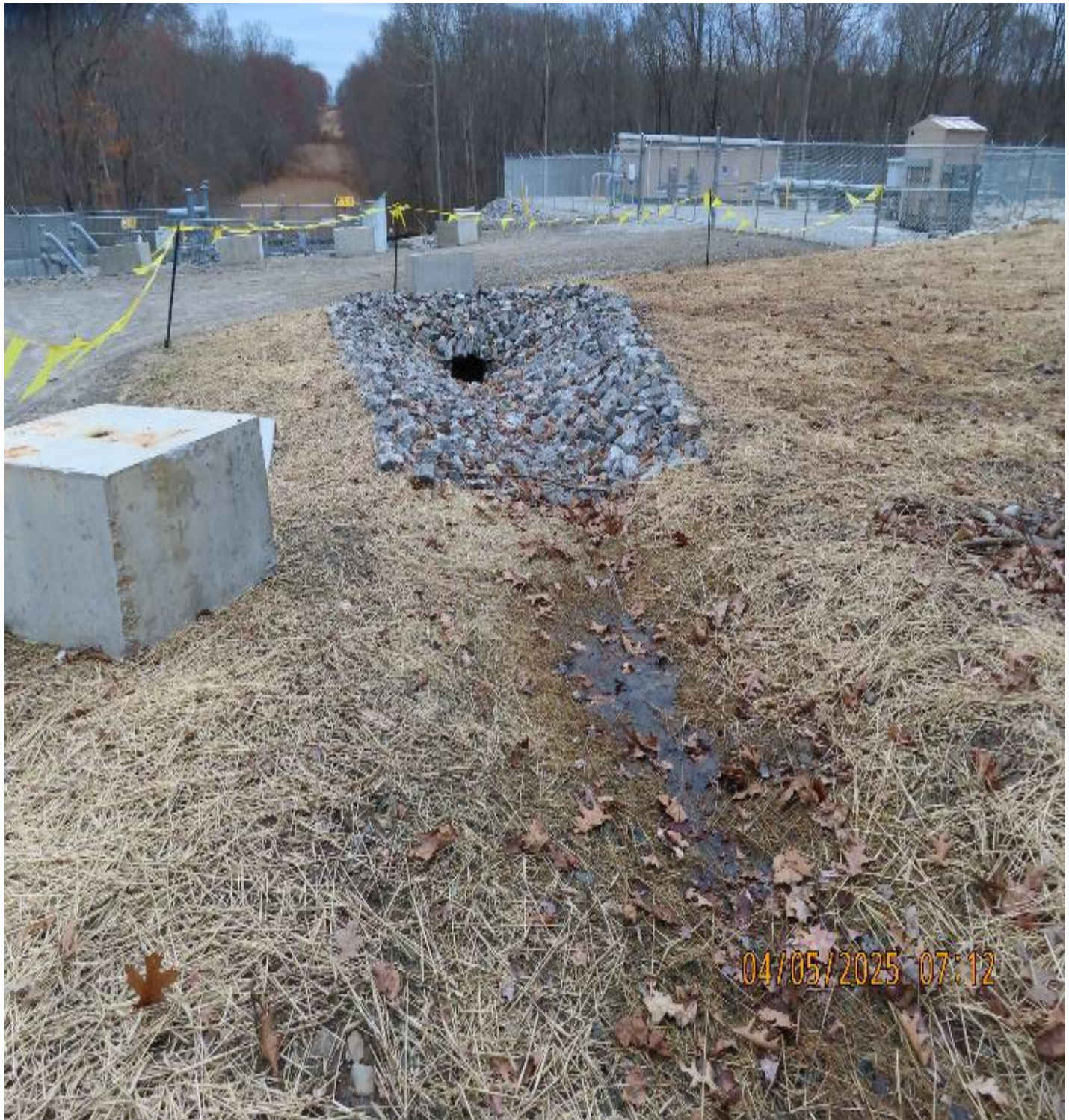
Photo 4: View (looking northeast) of drainage swale and culvert at valve yard entrance.
