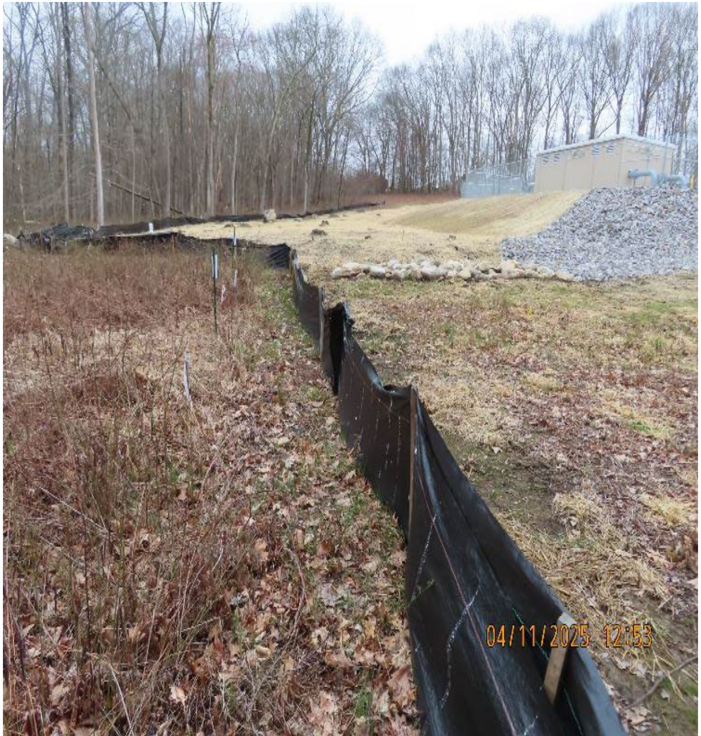
Photo 6: View (looking east) of silt fence along boundary of wetland W-CZ-01 and new regulation building in the background.
