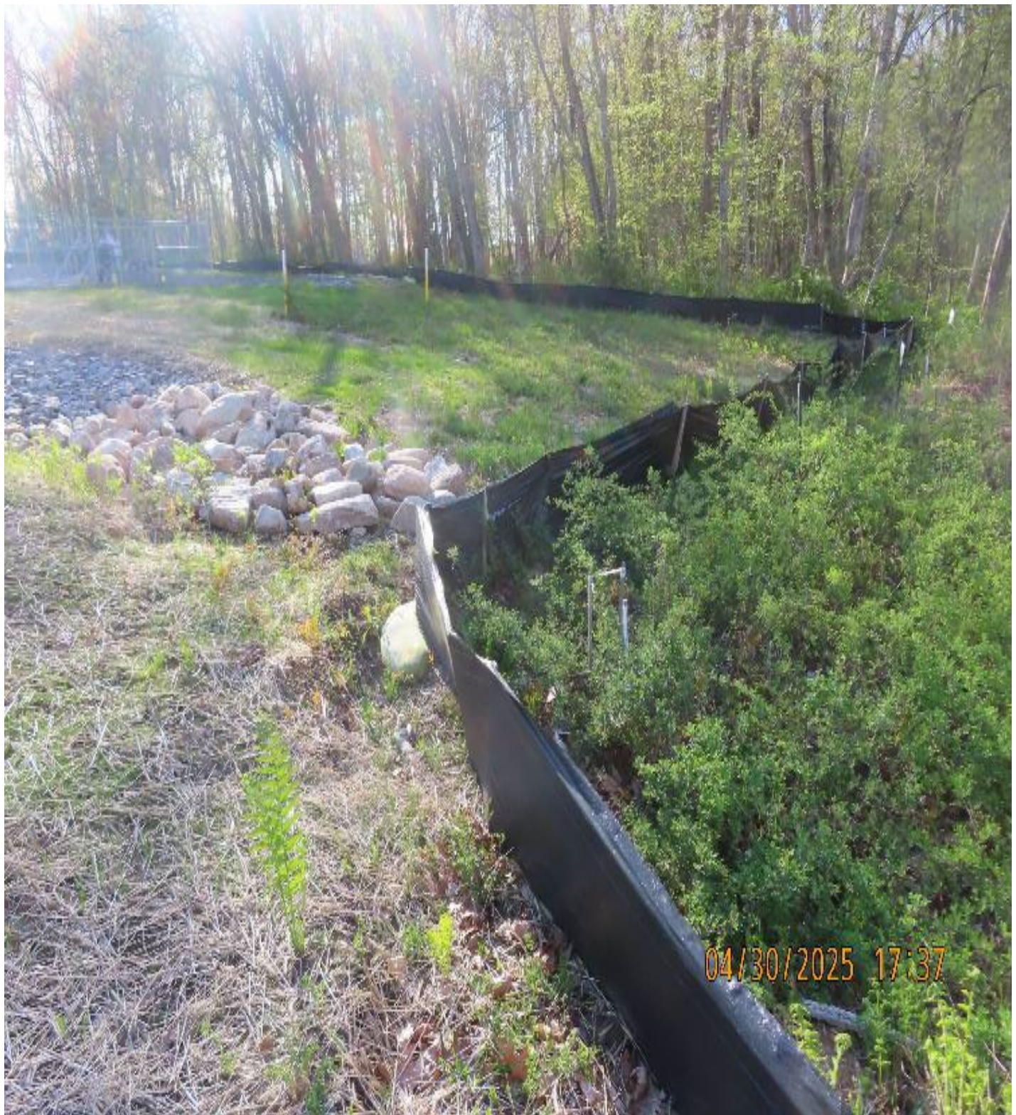
Photo 7: View (looking west) of silt fence and vegetative buffer along boundary with wetland W-CZ-01.
