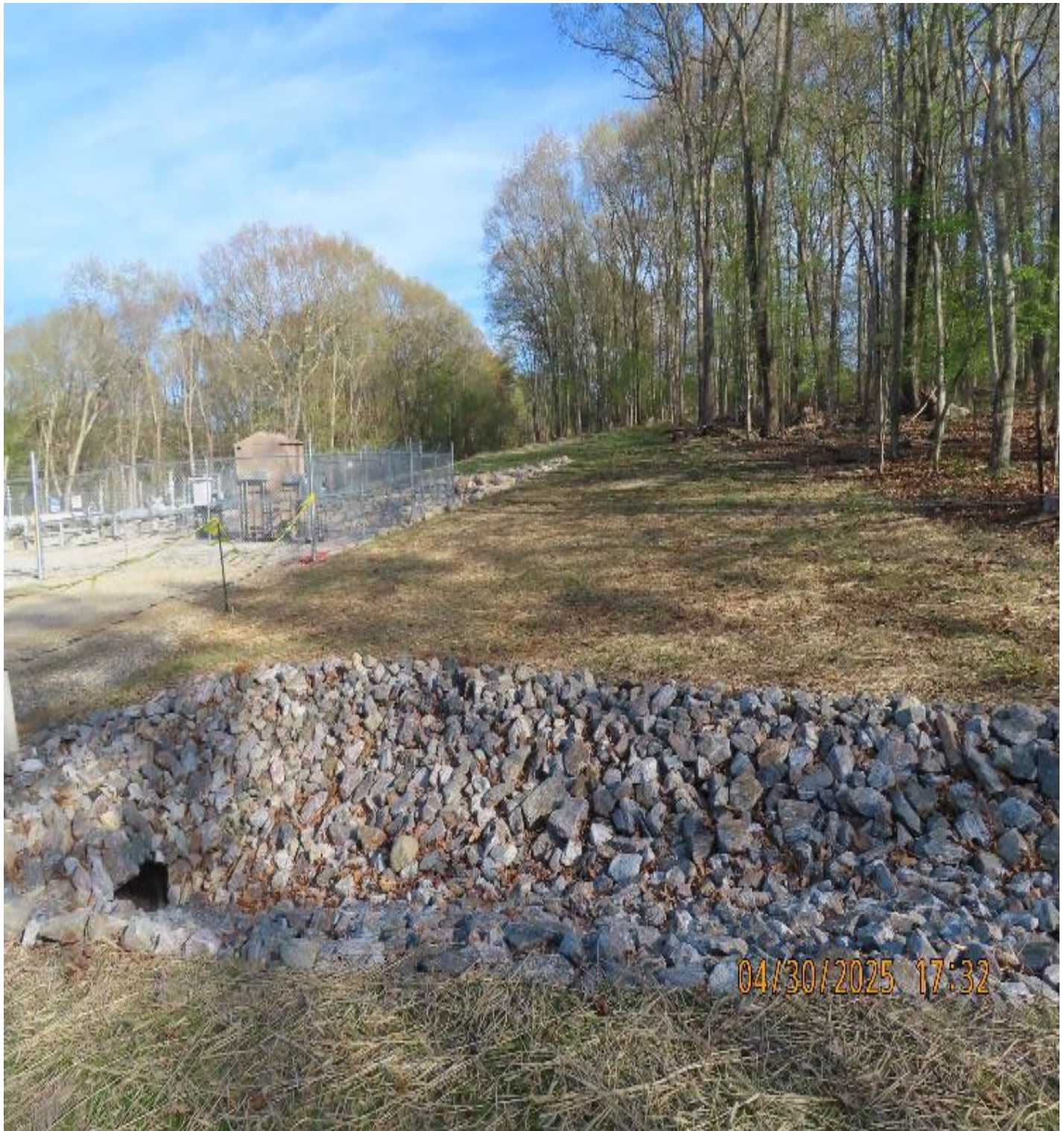
Photo 5: View (looking east) of stabilized drainage swale inlet to stormwater culvert near the valve yard.
